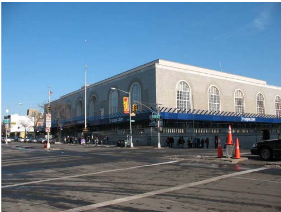
(9) View looking northeast to the former Bronx Central Annex (Resource 9) of the United States Post Office, 558 Grand Concourse.
