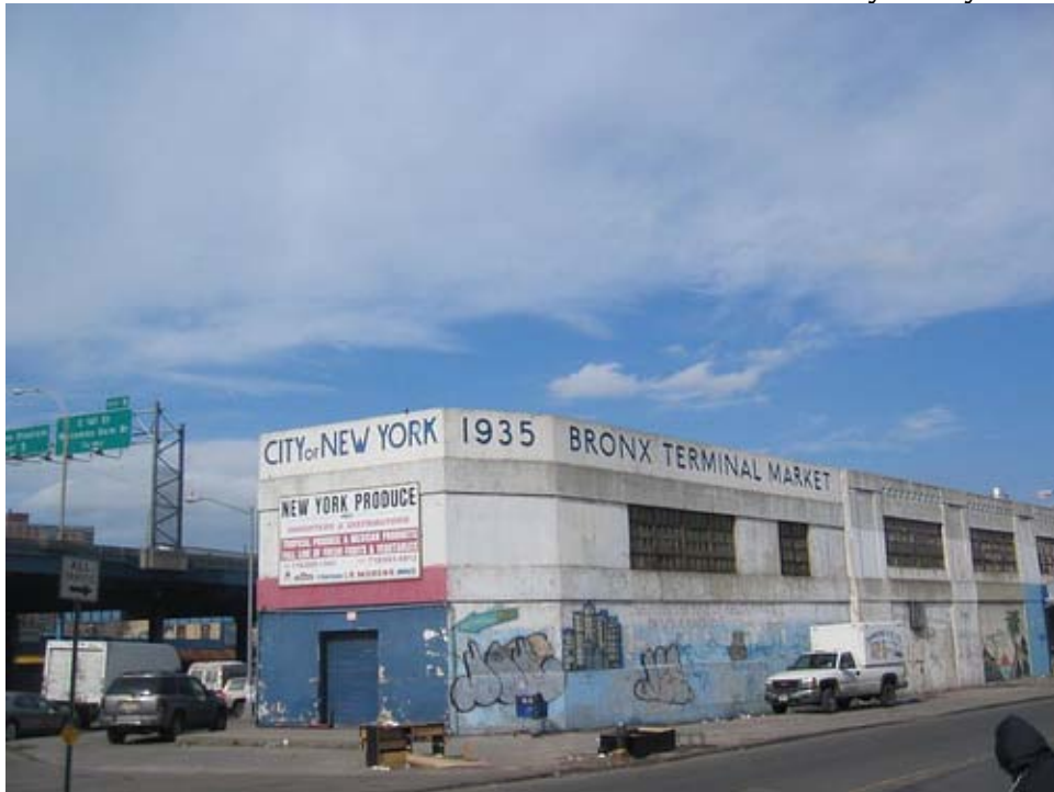
(12) View looking north-northwest to Building D (Resource 12), at the intersection of River Avenue and East 149 th Street, a remaining structure of the former Bronx Terminal Market.
