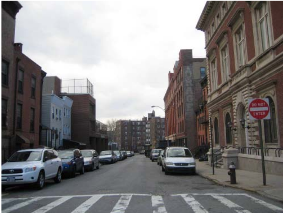
(3) East 140 th Street viewed looking east from Alexander Avenue.
