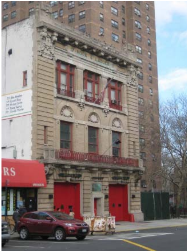
(24) Firehouse Hook and Ladder (Resource 24), looking north from E 143 rd Street.
