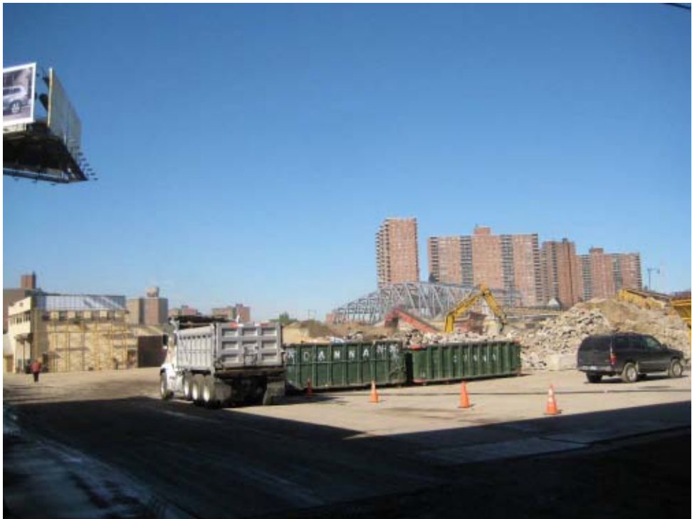
(6) Concrete manufacturing facility south of East 149 th Street viewed looking west from Exterior Street.
