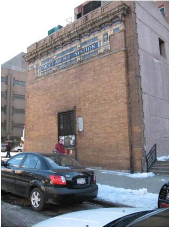
(3) View looking southeast to the Mott Avenue Control House (Resource 3) at the southwest corner of East 149 th Street and Grand Concourse.
