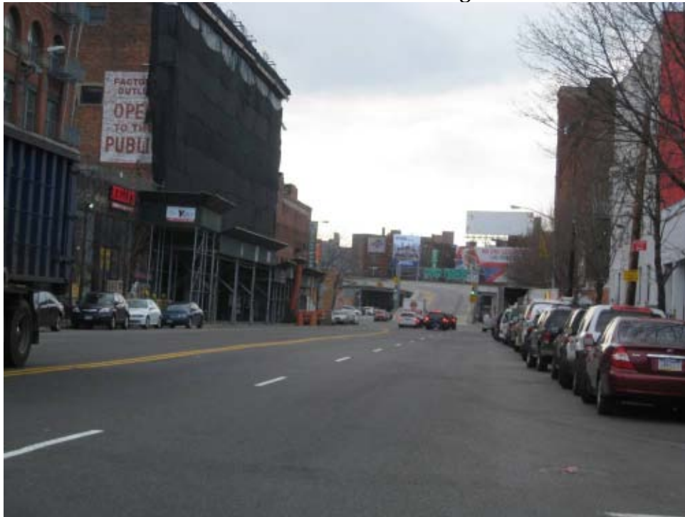
(3) Bruckner Boulevard and Third Avenue Bridge viewed looking west from Alexander Avenue.
