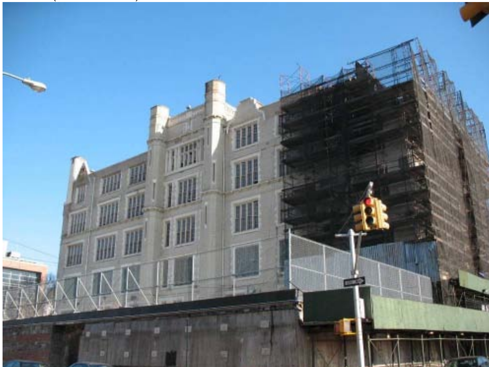
(2) View looking northeast to Public School 31 (Resource 2), 425 Grand Concourse.
