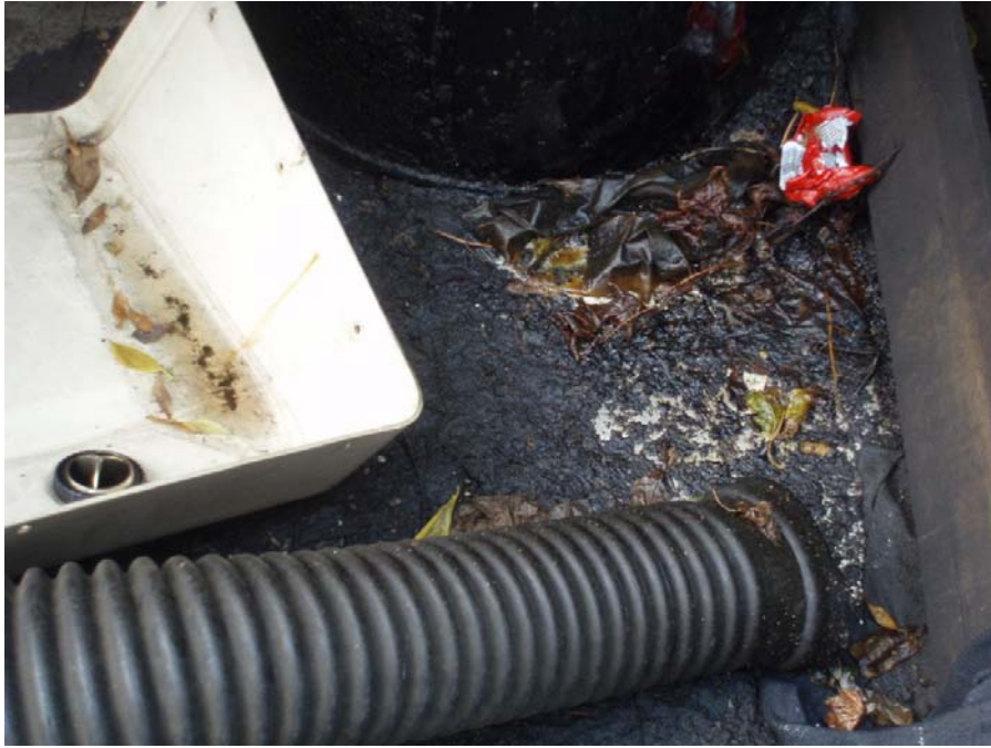
Photograph 23 – Lot 100: Black Material on Ground Beneath Drum
