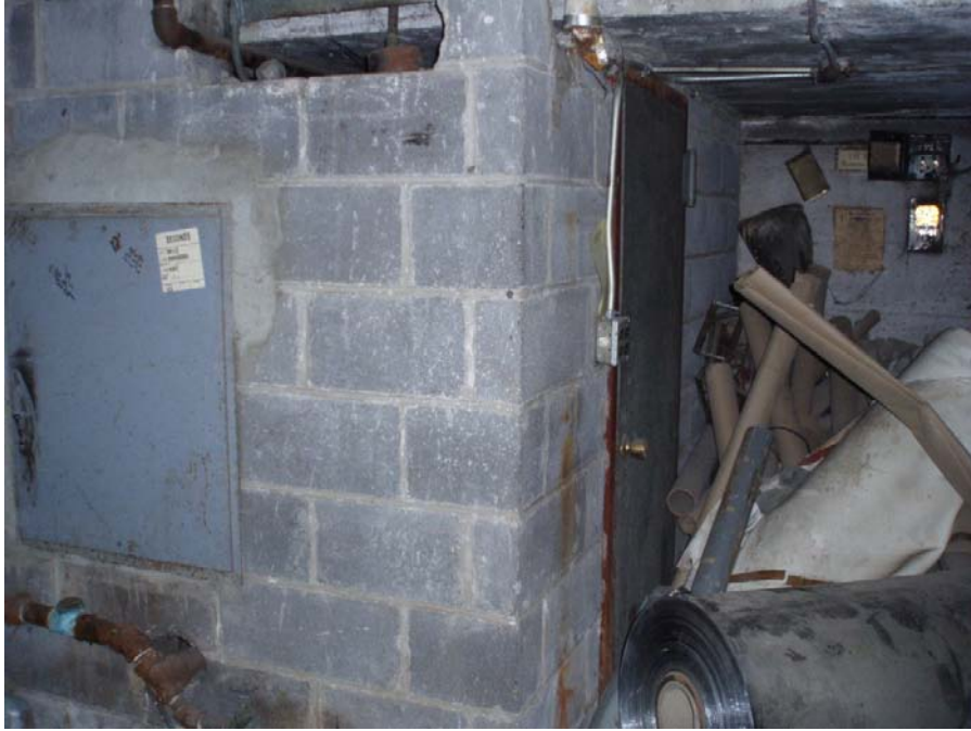
Photograph 39 – Lot 107: Concrete Block Furnace Room
