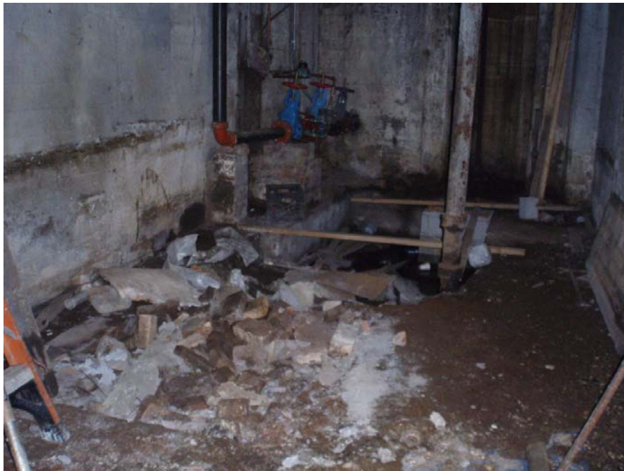
Photograph 32 – Lot 103: Former Boiler Room in Basement
