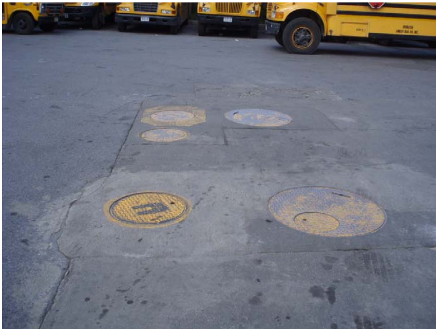
Photograph 16 – Lot 100: Location of Underground Storage Tanks
