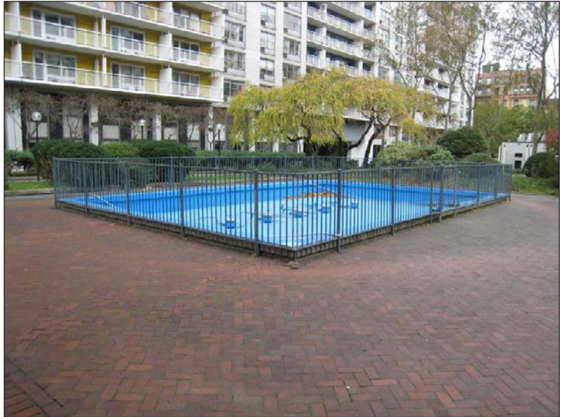
Washington Square Village Courtyard— View southwest to fountain 38
