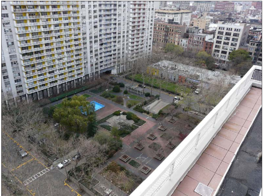
Washington Square Village Courtyard— 18 Aerial view southwest across the landscaped plaza toward the South Building
