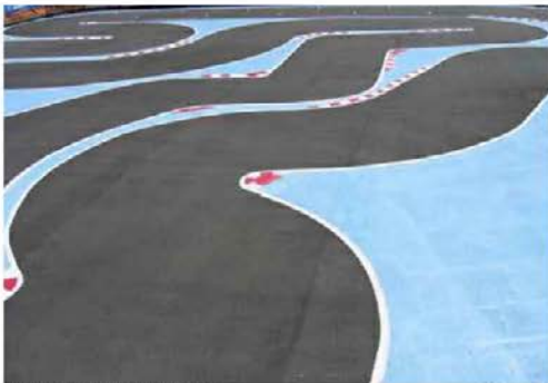
Printed Pavement Over Permeable Asphalt
