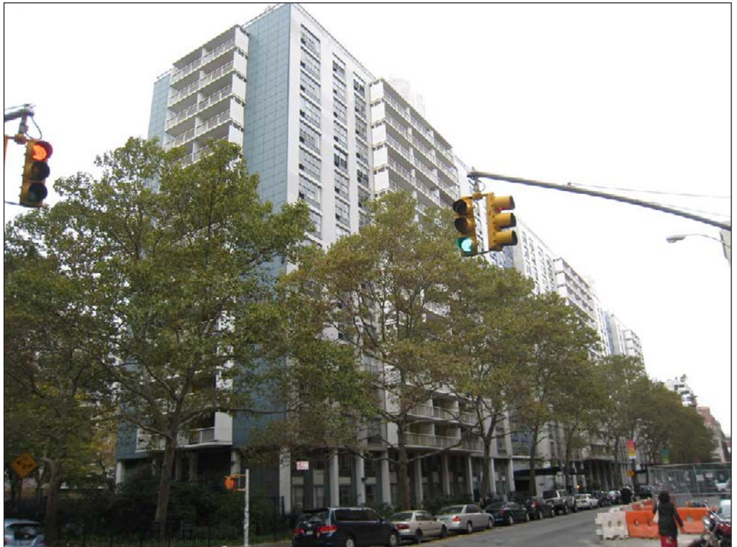
View southwest to Washington Square Village North Building—North facade 7
