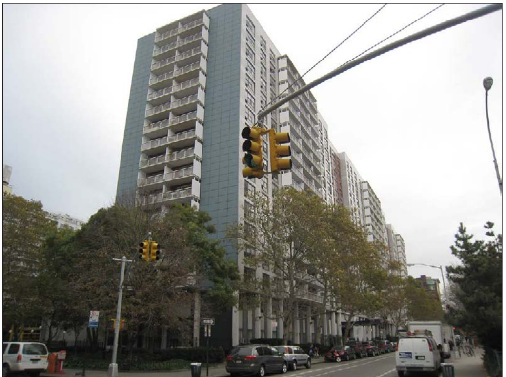
View northeast to Washington Square Village South Building—South facade 2
