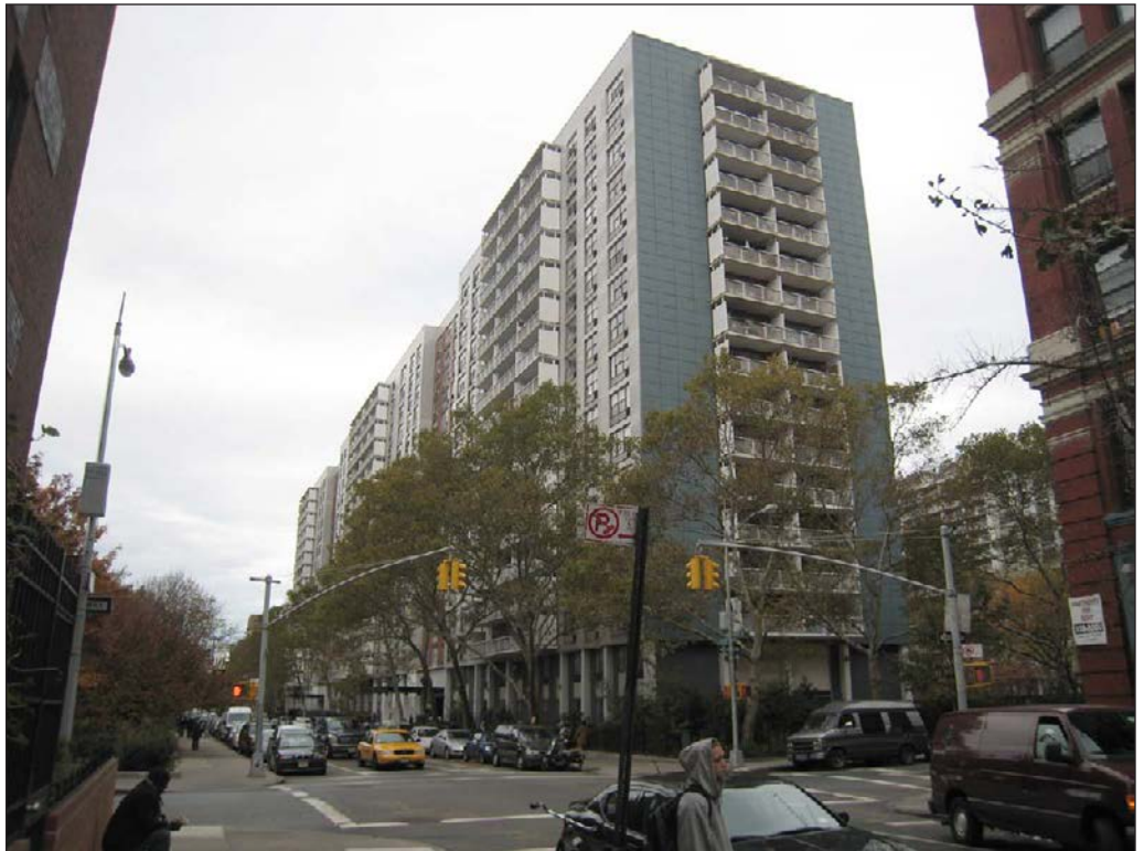
View northwest to Washington Square Village South Building—South facade 1
