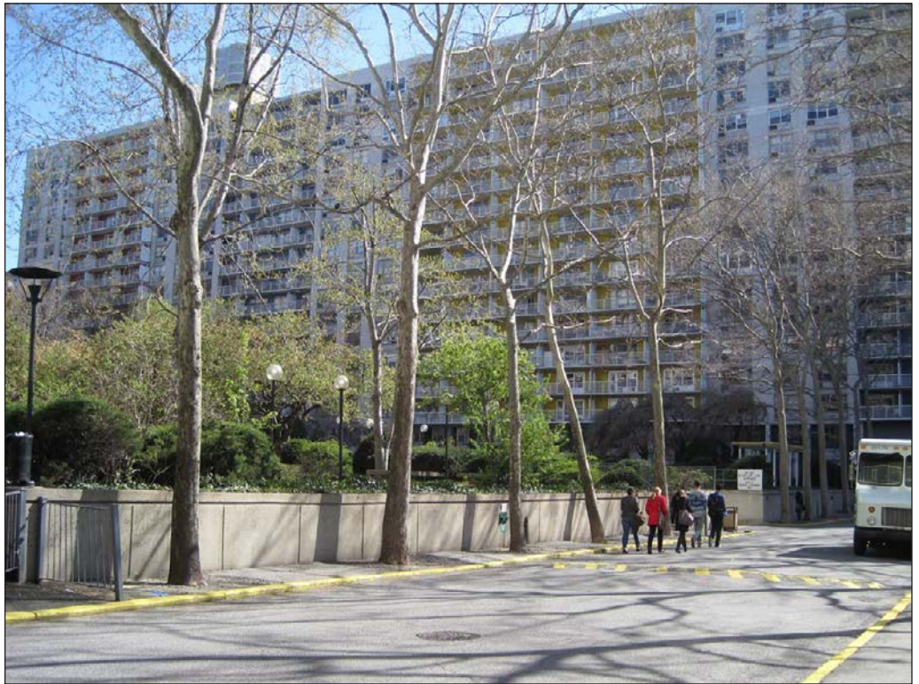
Washington Square Village Courtyard - View northwest on the Greene Street Driveway 27 toward the landscaped plaza
