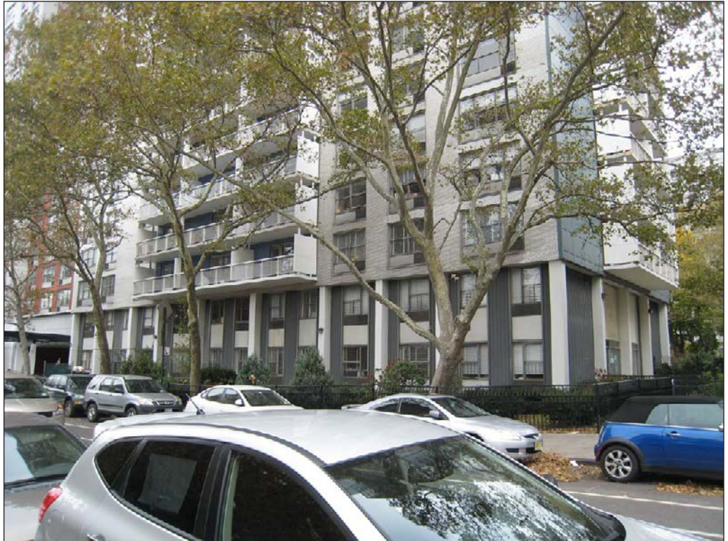
Washington Square Village South Building—South facade's lower floors 3
