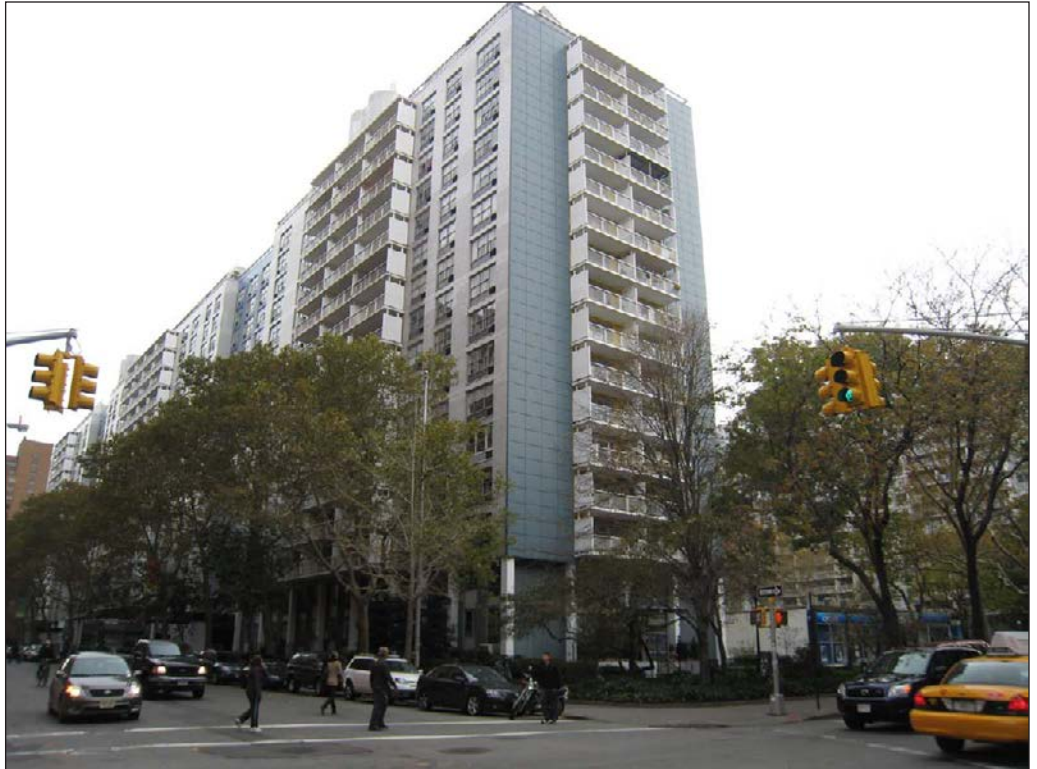
View southeast to Washington Square Village North Building—North facade 6
