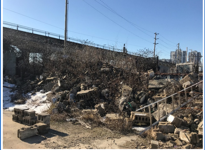
Photo 2: Construction debris (typical).
