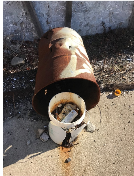
Photo 6: Rusted, empty 55-gallon drum.
