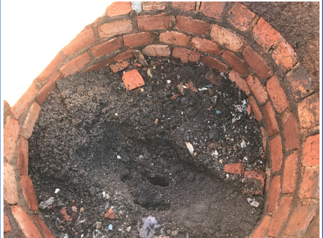
Photo 10: Interior view of the subsurface structure.
