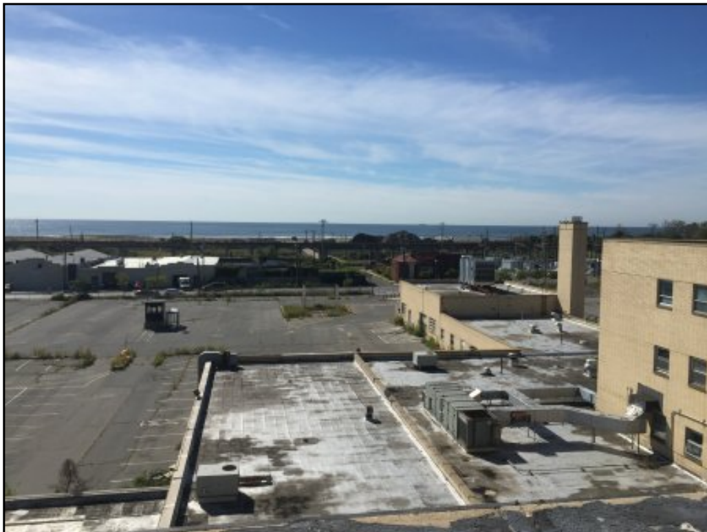
View of easterly portion of parking area (facing south) adjacent to furnace room. Suspected 10,000-gallon USTs located beneath parking area between guard shed and overhead doors at furnace room.
