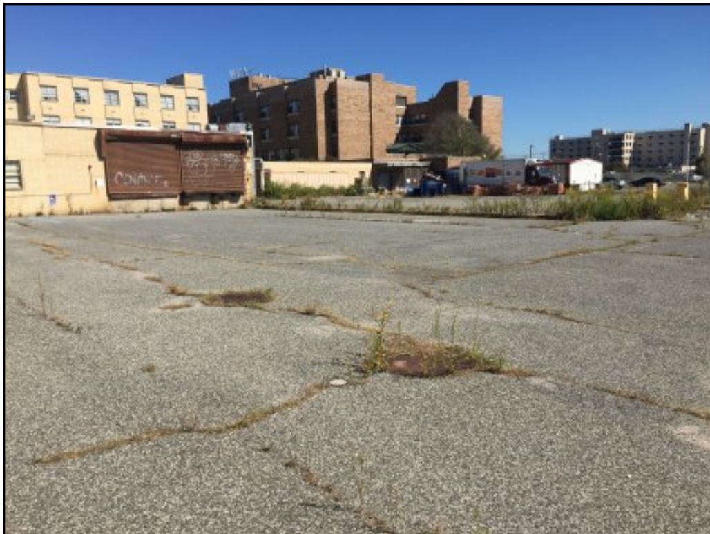
Two flush-to-grade manholes, consistent with fuel storage tanks, located immediately east of furnace room. View facing northeast.
