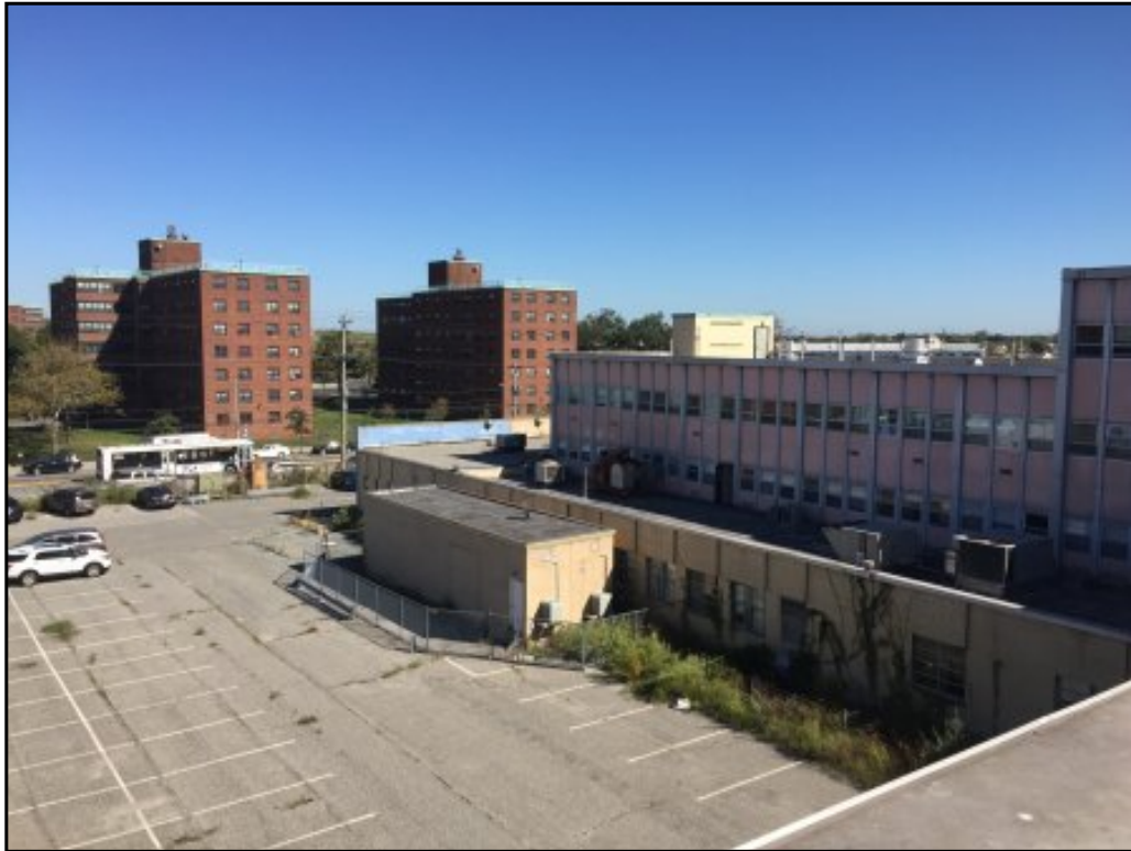
View of adjoining properties to the north, and the northerly portion of the eastern structure.
