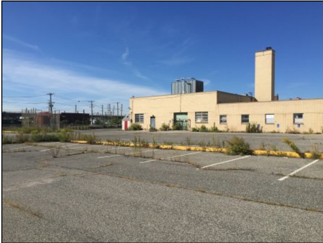
View of overhead door and entrances to furnace room. View facing southwest.
