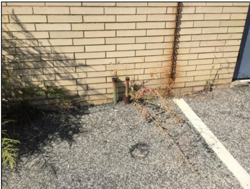
Suspected fuel tank fill and vent piping
