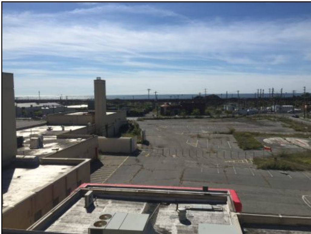
View of parking area along the westerly side of furnace room, note the 5,000-gallon AST located at the southerly extent of the furnace room.
