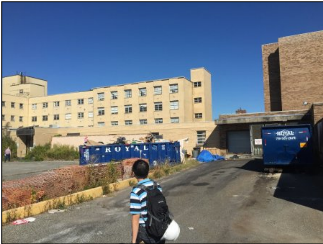
View of southeastern portion of eastern building. View facing north.
