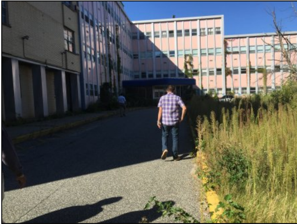
Front entrance to hospital (eastern building)
