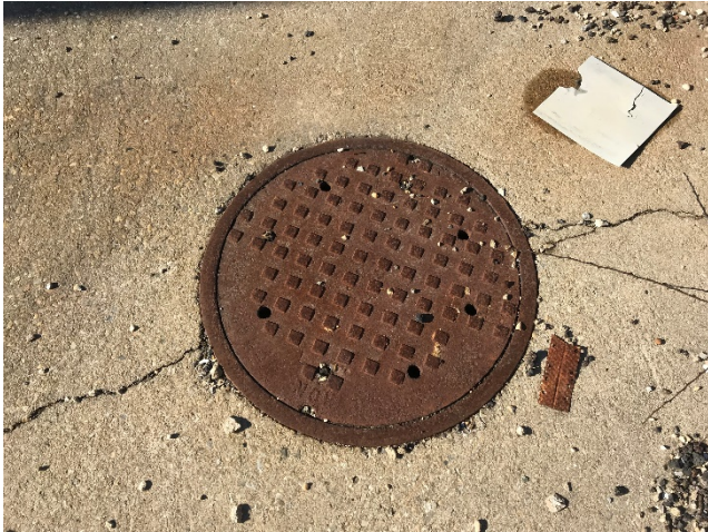
Photo 9: Subsurface structure cover in concrete-paved area (typical).
