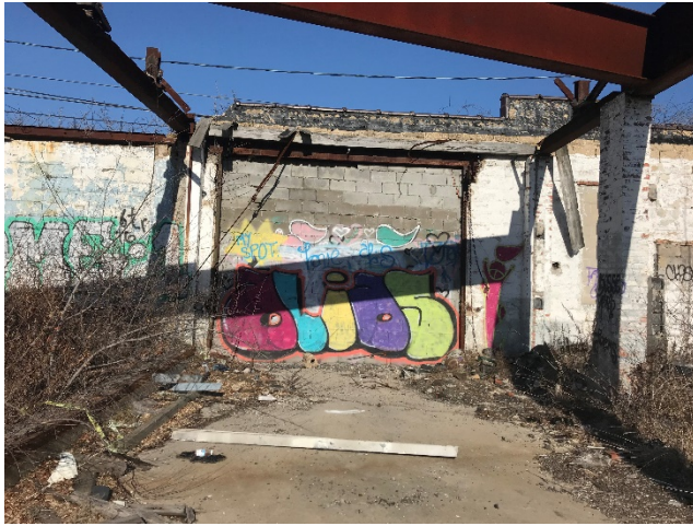
Photo 5: Former garage door entrance/exit along Rockaway Beach Boulevard.
