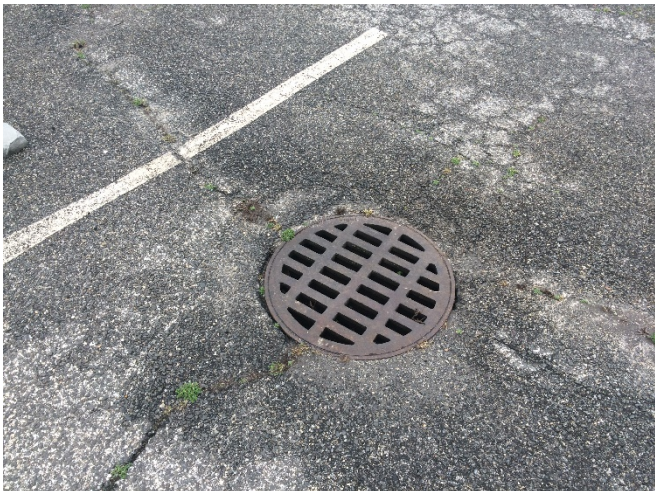
Photo #3 – Stormwater catch basin (typical).
