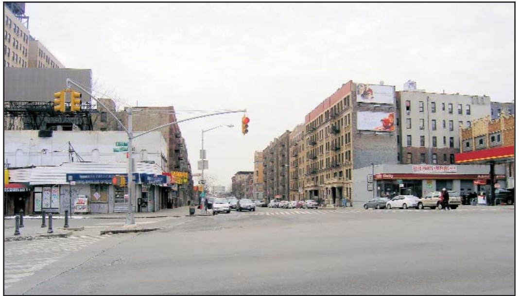
View from corner of W. 155th Street and St. Nicholas Place, looking south. Gas station adjacent to the Proposed Development Site is on the corner to the right, existing garage visible in the far right center.
