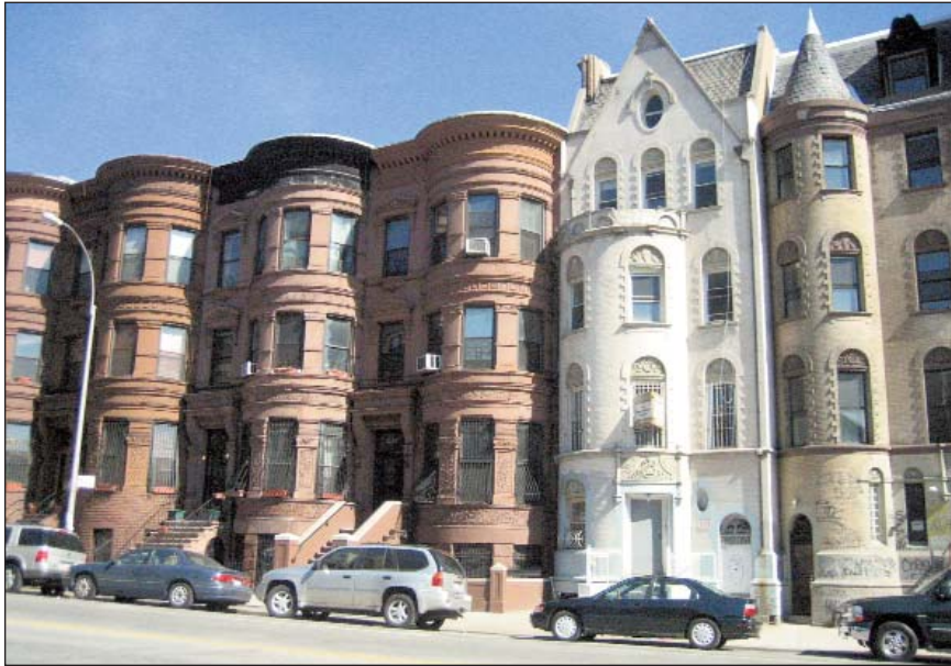
Above: View of eastern blockfront of St. Nicholas Avenue between W. 152nd and W. 153rd Streets. (S/NR district and LPC Hamilton Heights/Sugar Hill Northwest HD)
