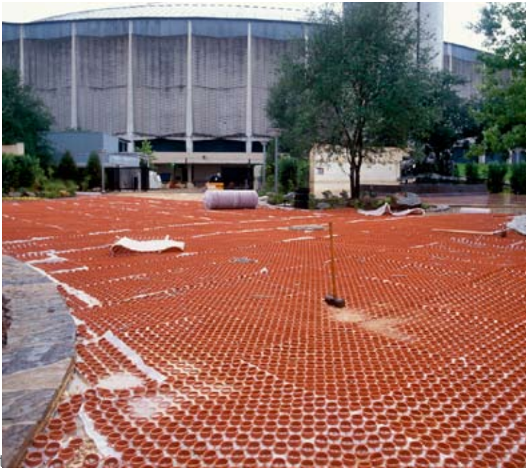
Reinforced grass pavers, shown here at the Reliant Stadium in Houston, TX, rely on a hidden structure of plastic cells in which grass is planted. The plastic cells keep the grass from being compacted, even when cars are parked on top. Image used with permission of Invisible Structures, Inc.
