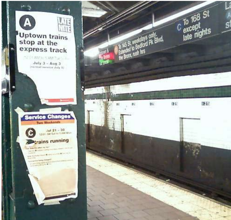
Ripped service announcement signs at 125th Street A/C/D/B platform. NYC Dept. City Planning
