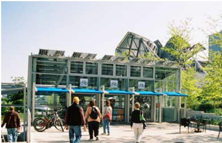
The McDonalds Cycle Center in downtown Chicago, offers amenities such as lockers and showers and a café. Image used with permission of McDonalds Cycle Center
