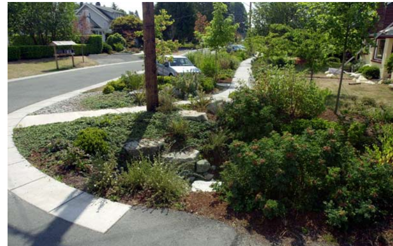
Seattle SEA Streets, built primarily in residential neighborhoods, reduce rain run-off and flooding with bio-swales and improved street design. Image source: NYC Dept. City Planning
