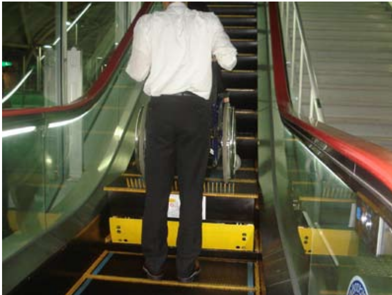
Wheelchairs are secured by a guardrail in the back and an attendant who holds the wheelchair in place. Image used with permission of Kansai International Airport (KIAC).
