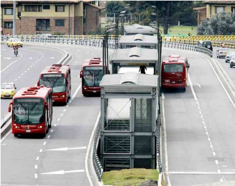
A Transmilenio station in Bogotá, Colombia. The double lane designated right-of-way allows for express and local service, while the physical barrier between the bus lanes and regular traffic reduce the need for enforcement.
