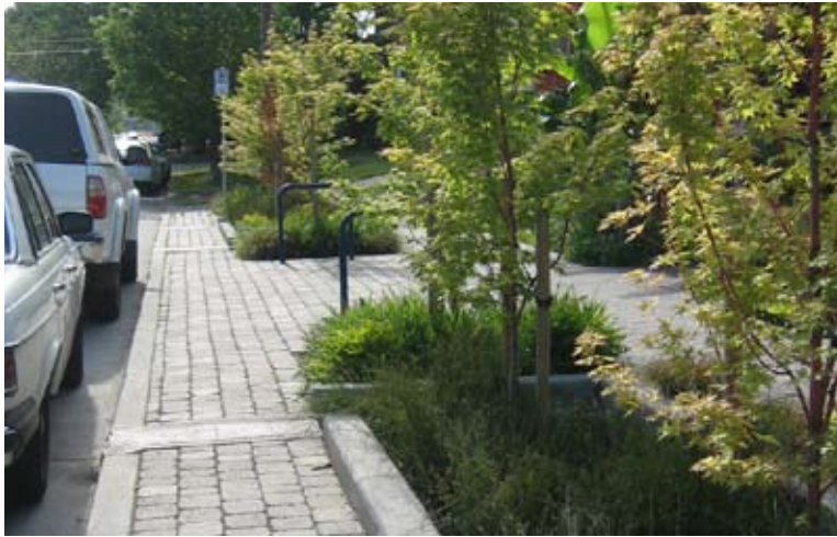
A narrow strip of porous pavers provides room for passengers to exit from their cars. The 12" wide, ADA accessible metal grate in the foreground covers the inlet by which rain run-off enters the planter. Image source: NYC Dept. City Planning
