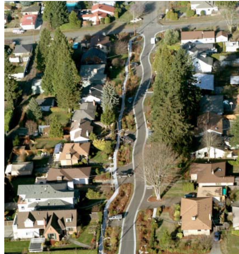
The SEA Street pilot (NW 117th and NW 120th Street on 2nd Avenue). The slight curves in the roadway slow the rain run-off as it flows down the street. The SEA Street design also serves as a traffic calming device and added sidewalks to a neighborhood that previously lacked them. Images used with permission of Seattle Public Utilities.
