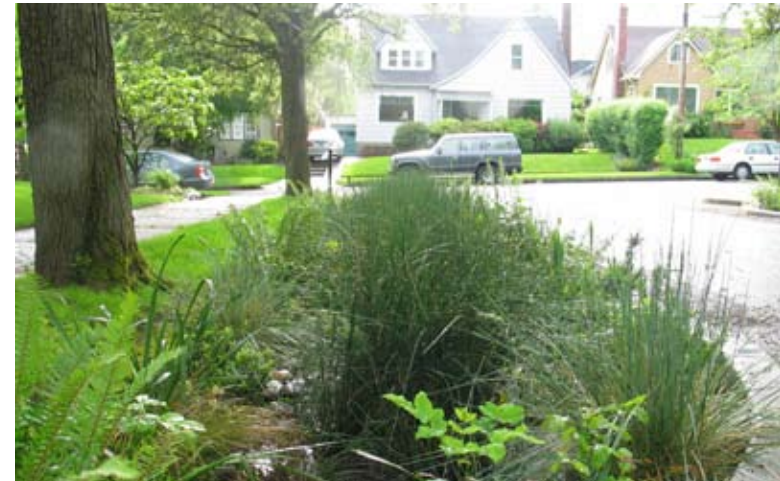
Portland's planted curb extensions enhance the aesthetics of the streetscape while reducing water run-off and flooding and calming traffic. Image used with permission of City of Portland Bureau of Environmental Services.
