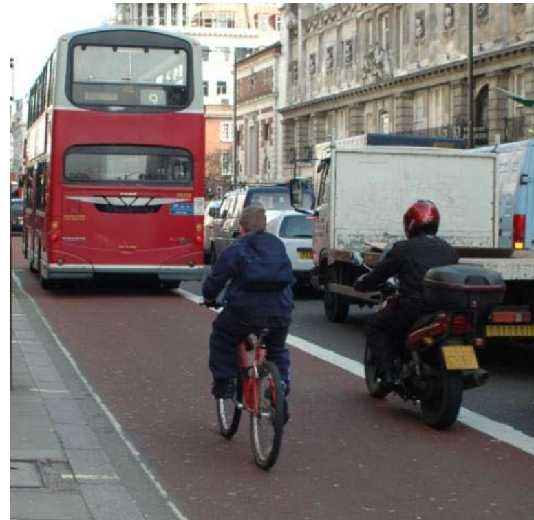
Bicycles, motorcycles and buses share a non-physically separated bus right-of-way in London. The colored asphalt increases the visibility of the right-of-way. Crown copyright, from DfT TAL207, reproduced with permission.
