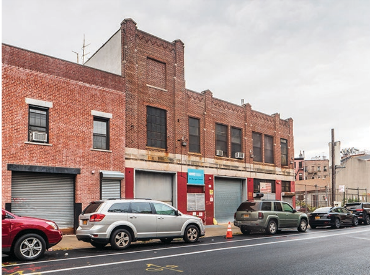
View of 516 Bergen St, looking south, between Carlton Ave and 6th Ave
