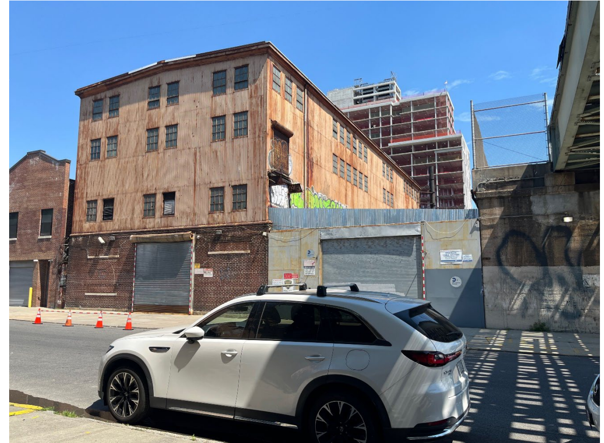
View of the MTA Cable repair and storage buildings, looking north from Pacific St under the elevated rail
