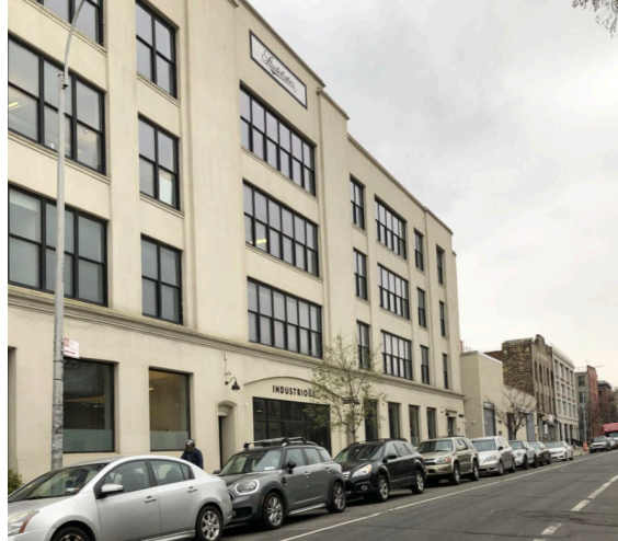
Offices at 1000 Dean St
