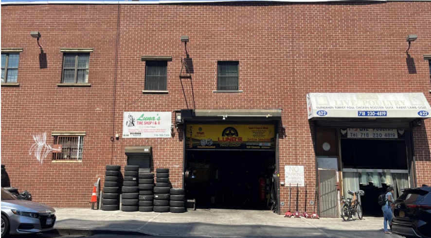
Auto repair on Classon Ave and Dean St
