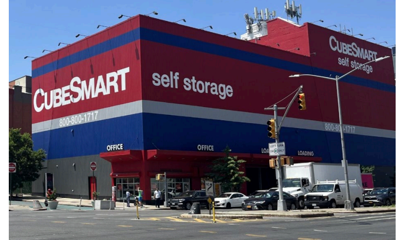
Self-storage along Atlantic Ave and Underhill Ave
