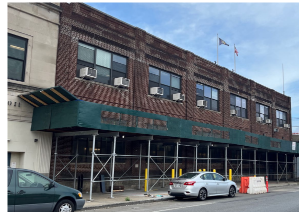
View of the MTA Cable repair and storage buildings, looking south from Atlantic Avenue
