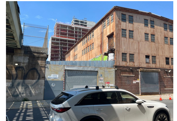
View of the MTA Cable repair and storage buildings, looking north from Pacific St under the elevated rail
