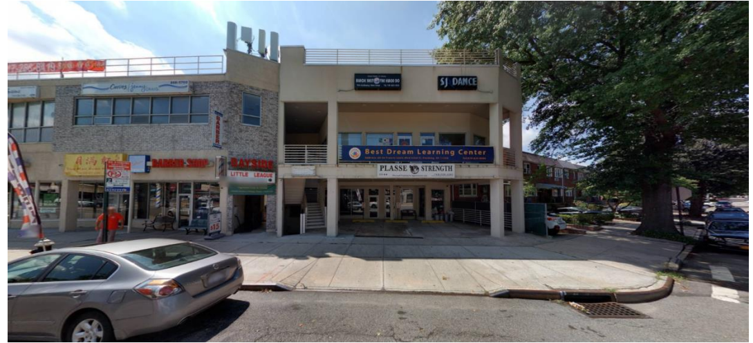
2 nd floor Community Facility in Queens. This space would not have been able to convert to commercial use.
