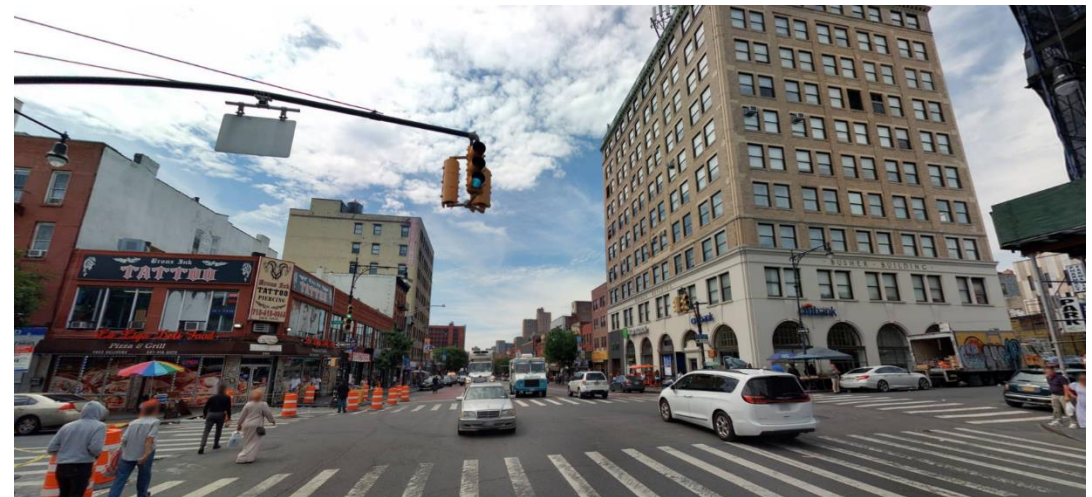
C4 district at the Hub, the Bronx, where zoning made it difficult to convert to residential
