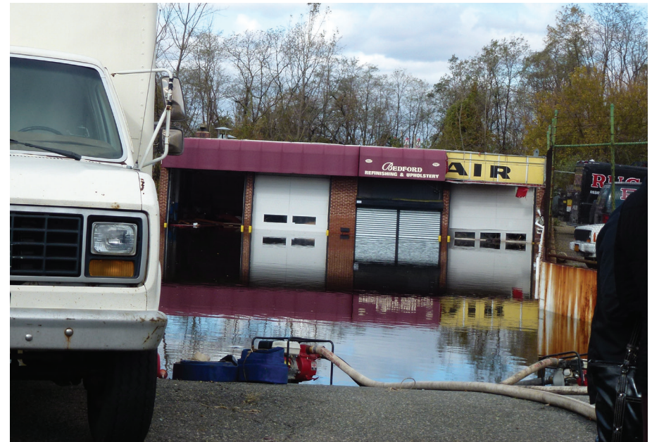
FIGURE 29: Standing water left in the aftermath of Hurricane Sandy along Richmond Terrace.
