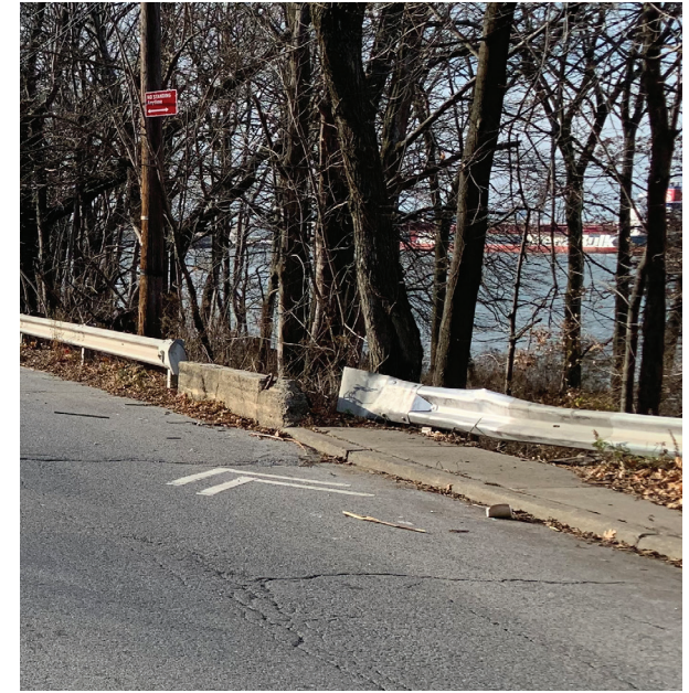
FIGURE 24: Worn shared lane marking on westbound Richmond Terrace at Snug Harbor.
