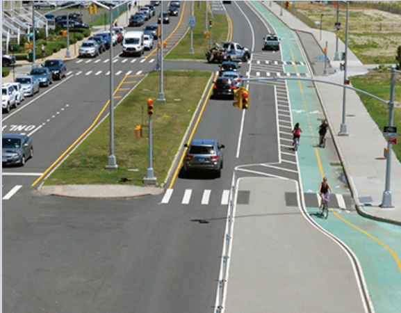
FIGURE 66: Shore Front Parkway, Queens Source: NYC DOT Street Design Manual
