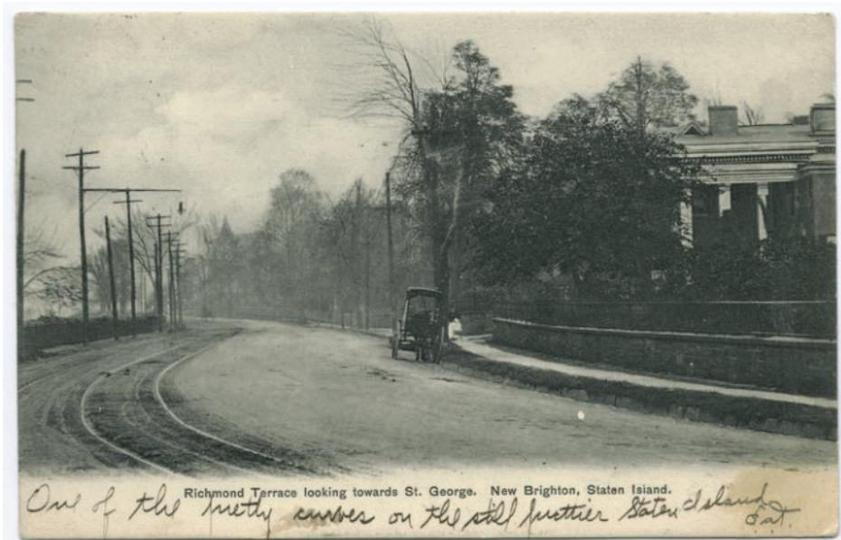
FIGURE 4: Historic Richmond Terrace, New Brighton, St. Horse and carriage parked in front of home, light poles, and trolley tracks.
