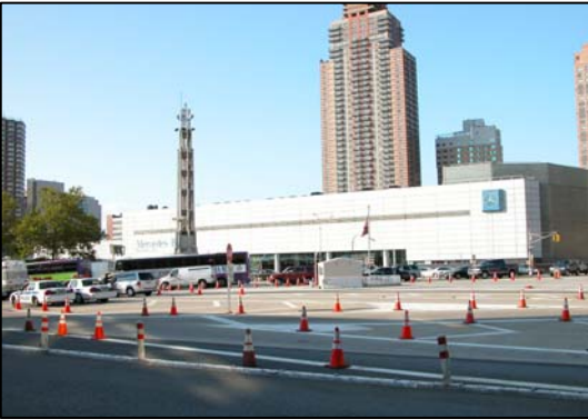
Existing conditions, looking north from 39 th Street across the Lincoln Tunnel entrance
