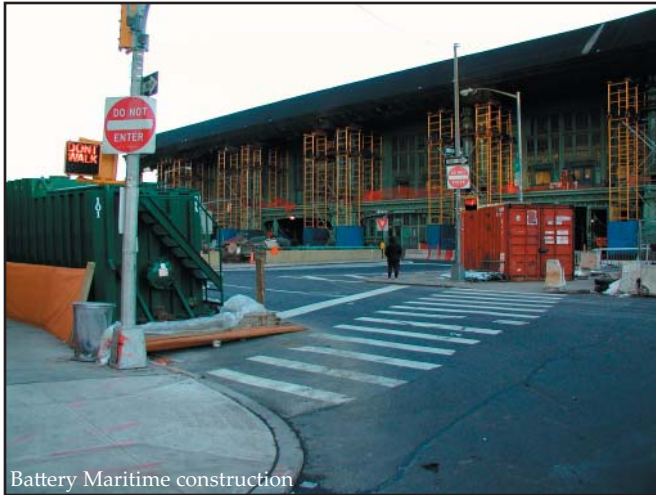
Battery Maritime construction
