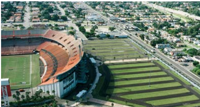
Orange Bowl - Reinforced Grass pavers, shown here at the Orange Bowl Stadium parking lot in Miami, FL, has dramatically increased the quality of the parking lot while also reducing the amount of water that storm drains and sewers must handle after rainstorms. Image used with permission of Invisible Structures, Inc.
