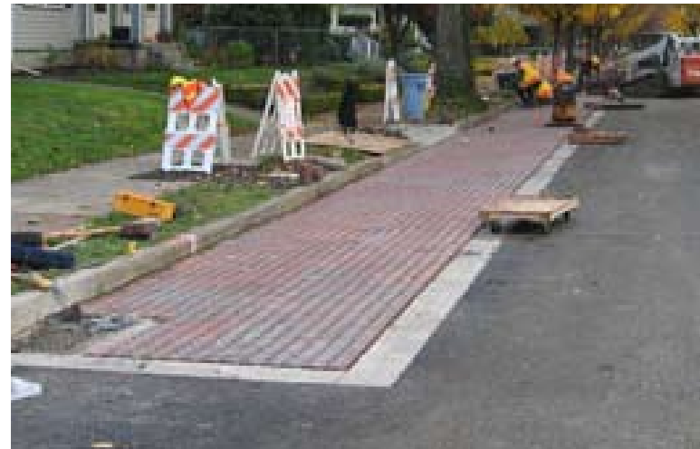
The Portland Bureau of Environmental Services is experimenting with pervious pavers and porous asphalt in residential neighborhoods. In this image, the pervious pavers serve a dual purpose, clearly marking the parking lane as well as reducing rain run-off and flooding. Image used with permission of City of Portland Bureau of Environmental Services.
