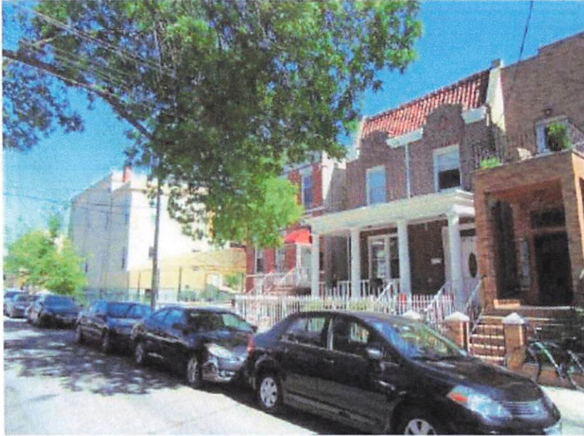
1. View of the Project Area facing northwest from 31st Drive.
