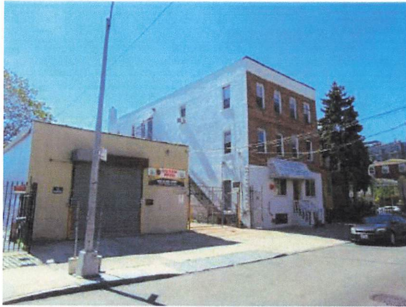
10. View of the Project Area facing south from 12th Street.
