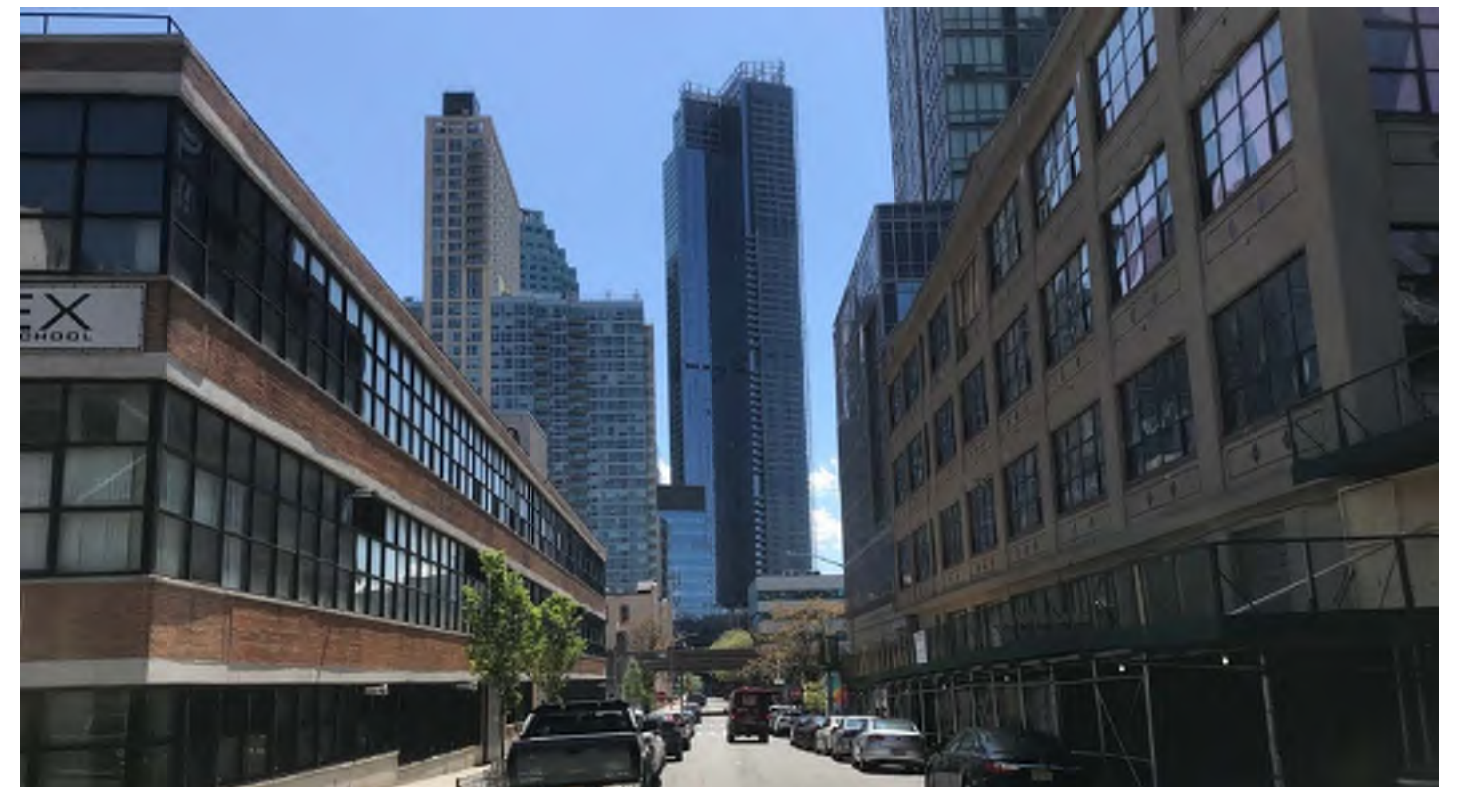
3. STREET VIEW FROM THE EAST CORNER SHOWING EXISTING BUILDING ALONG THE 24TH STREET
