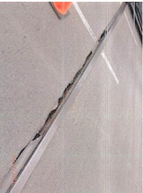
Replace Expansion Joints
