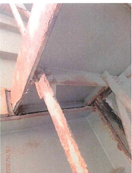
Repair Corroded Steel Superstructure
