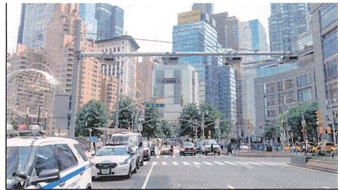
Congestion pricing cameras installed in Manhattan
