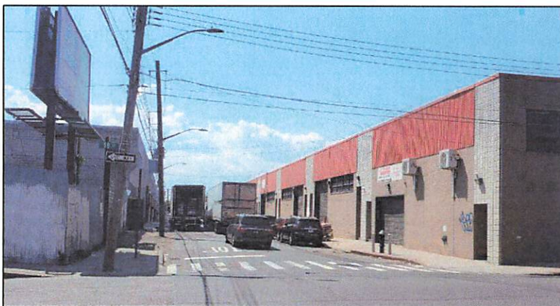
Before: 56 th Dr, 58 th St to Rust St St (QN)
