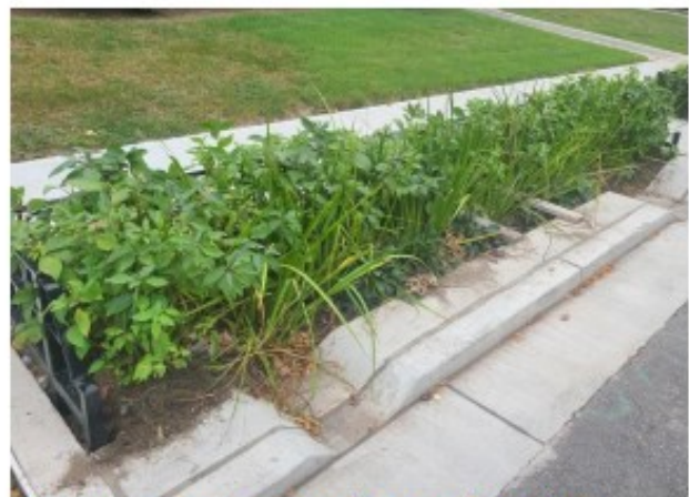
After Installing Bioswale on 185 th St bet. 69 th & 73 rd Ave
