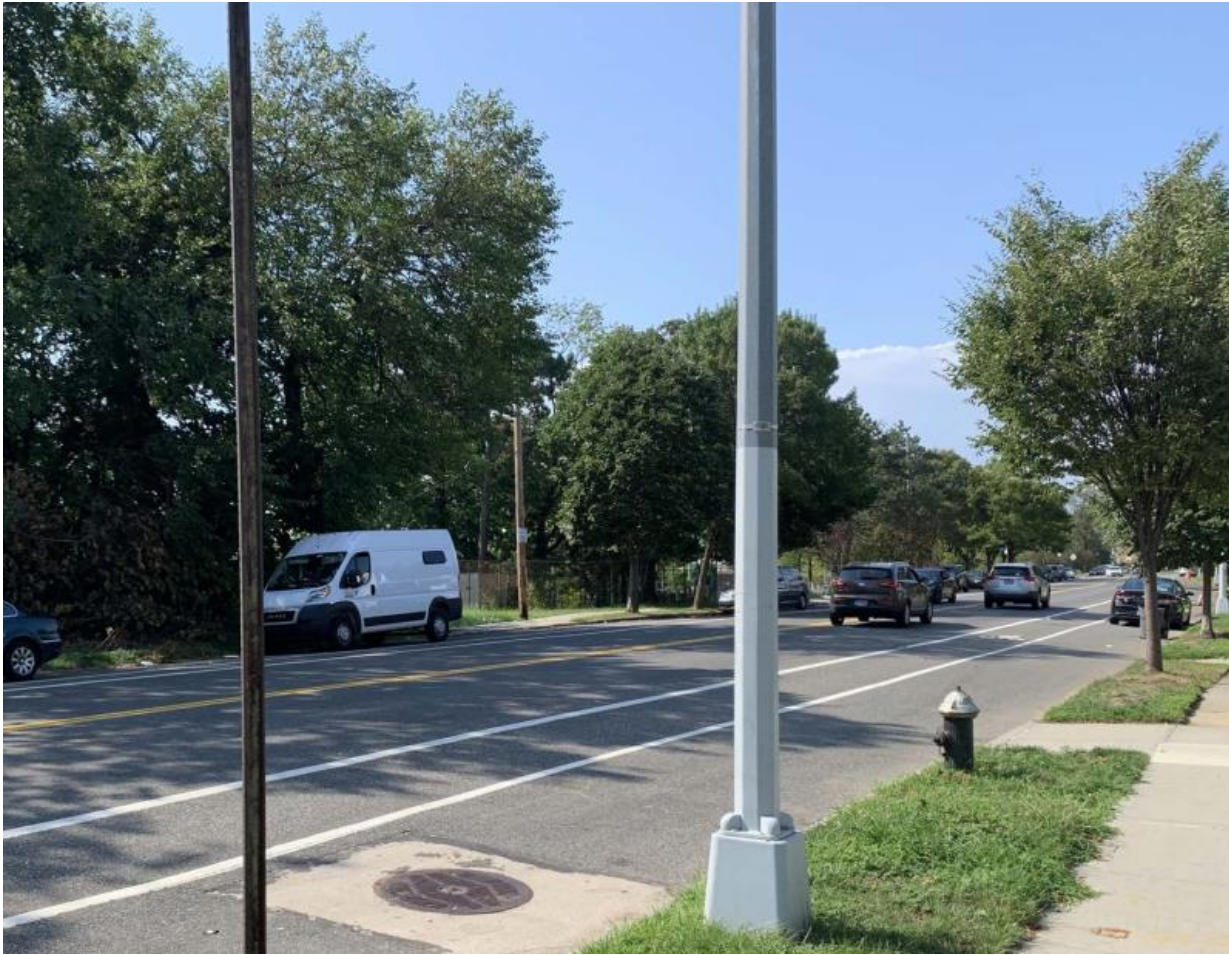
View of pump station from east side of Park Drive East
