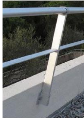
STAINLESS STEEL RAILING
