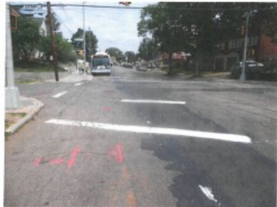
Completed road work on Homelawn and Highland Street
