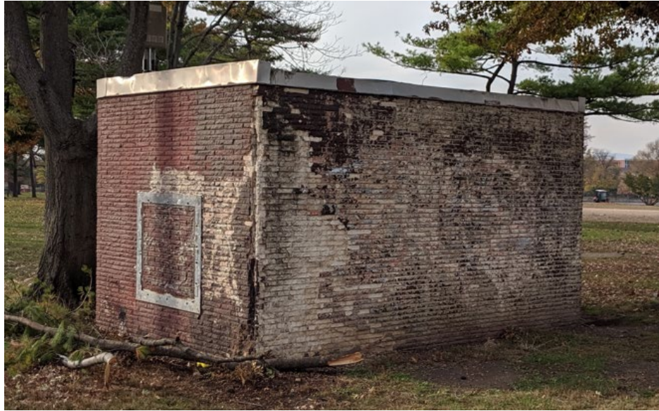
EXISTING VAULT K
