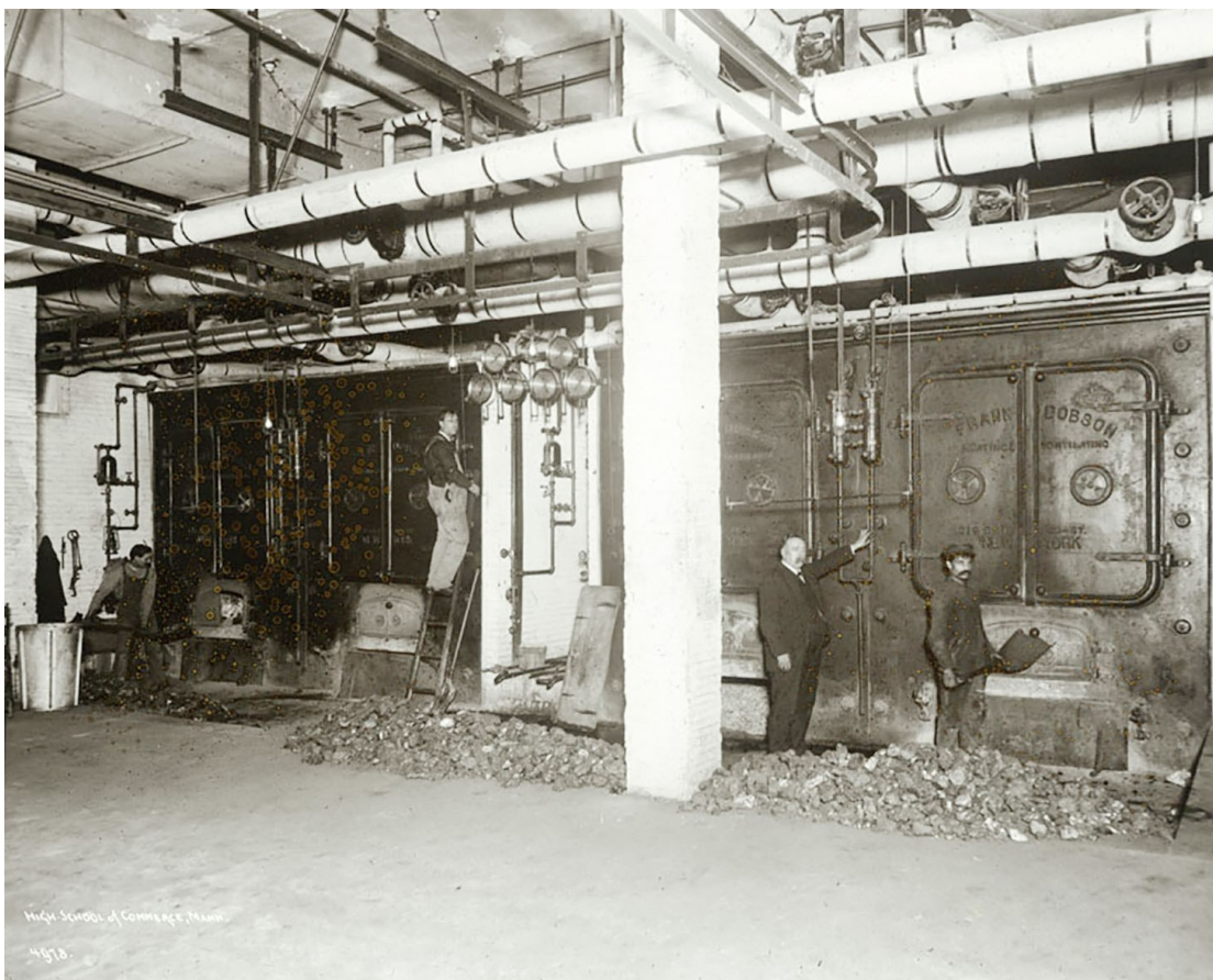
Undated photo of large coal heating apparatus in basement of High School of Commerce in Manhattan, with worker shoveling coal.
