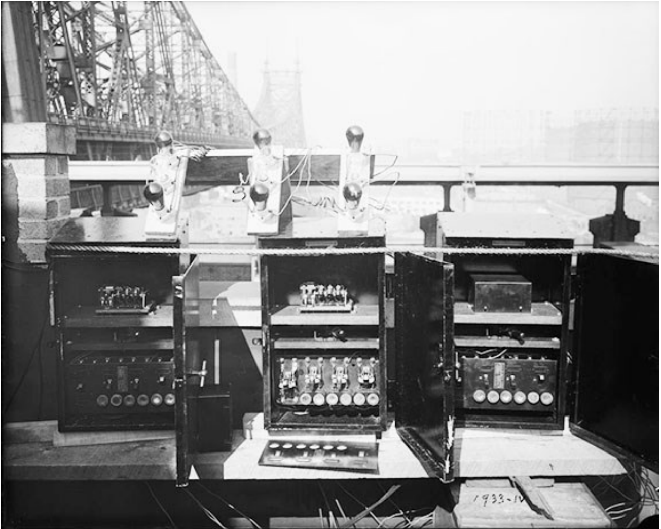
A September 1924 photo of the Queensboro Bridge experimental electric traffic light.
