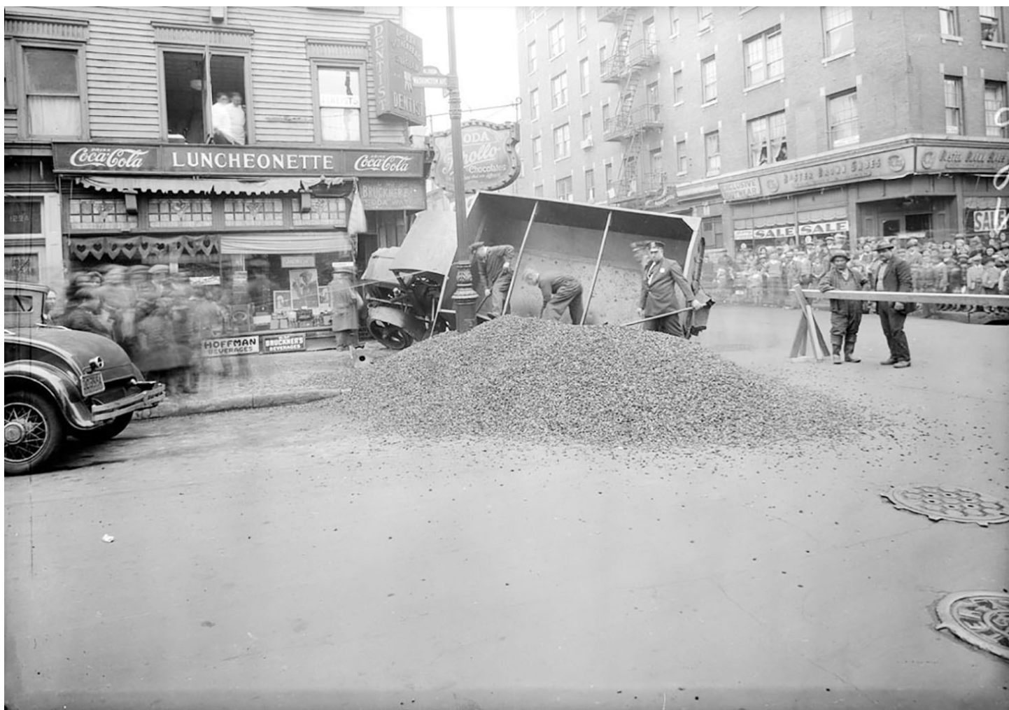
1931 photo of overturned coal truck on 169th Street & Washington Avenue, with coal scattered on street.
