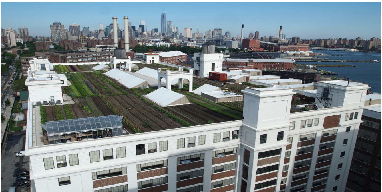
Rooftop garden at Brooklyn Navy Yard Photo credit: NYC Economic Development Corporation
