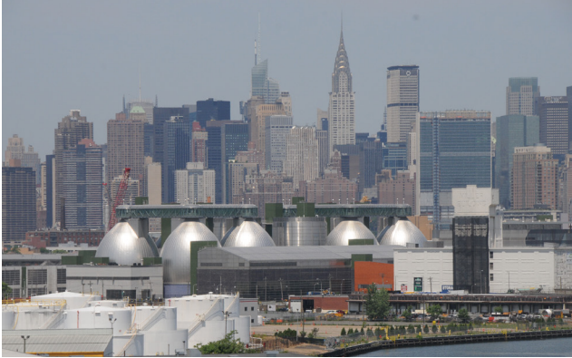
Anaerobic digestion facility at Newtown Creek WWTW Photo credit: NYC Department of Environmental Protection
