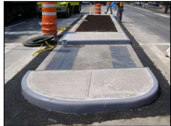
New pedestrian refuge island in south crosswalk
