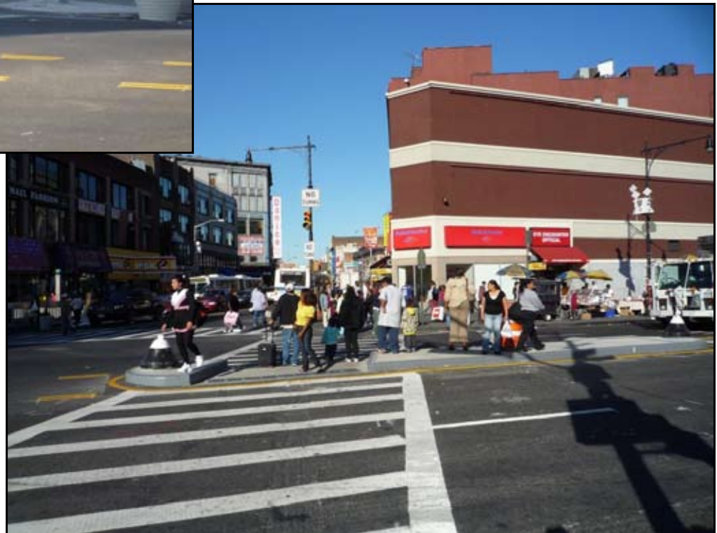
New pedestrian refuge island on East 149th Street at Third Avenue
