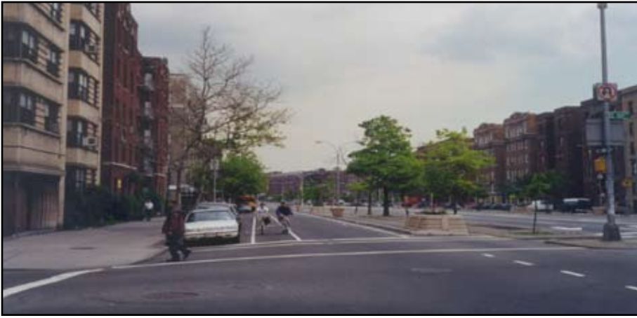
Grand Concourse/East 169 th Street Service Road after implementation of safety project with planters and bike lane
