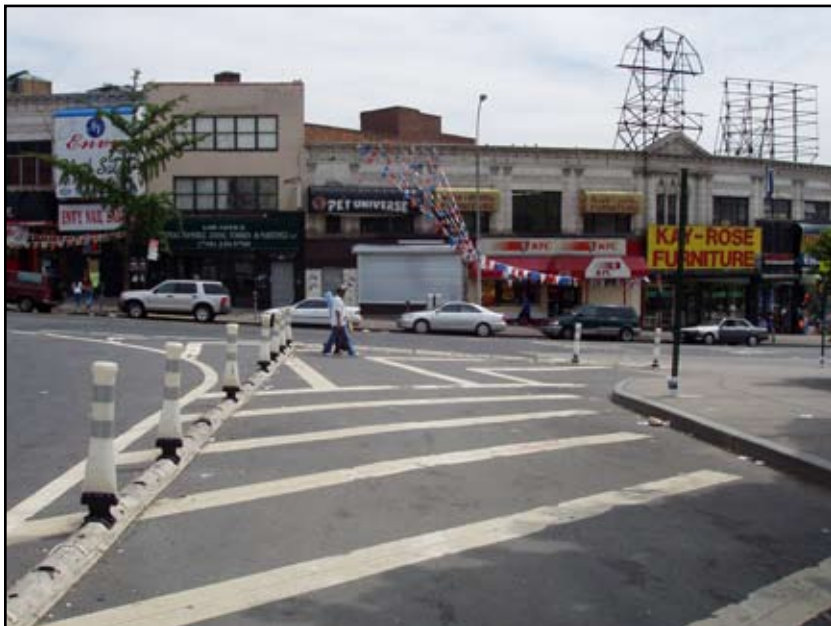
Flexible delineators and markings for increased pedestrian and vehicular safety
