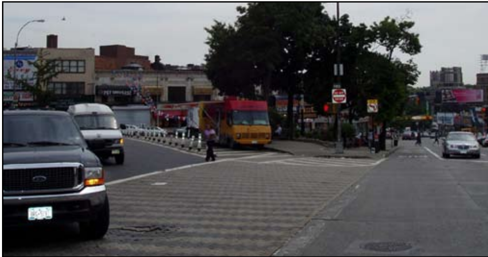
Detailed view of several of the improvements including one-way conversion of slip ramp, modified neckdown and flexible delineators surrounding the park
