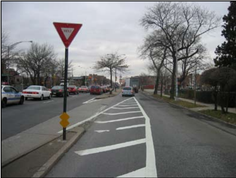
New markings to prevent illegal maneuvers between main line and service road
