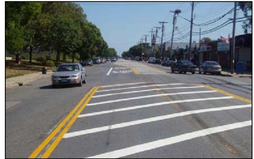
New painted center median and turning bays
