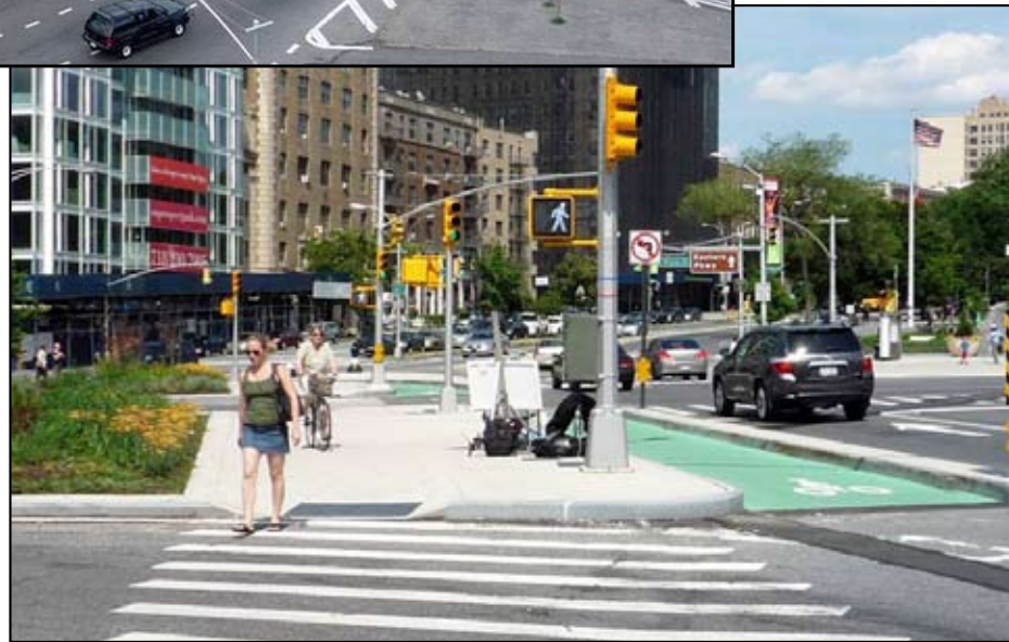
View of newly constructed Pedestrian Island with plantings, and Class 1 "green" bike path
