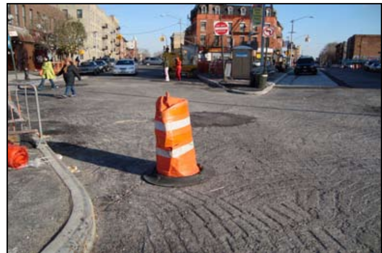
Permanent Treatments: Temporary treatments made permanent - currently under construction.
