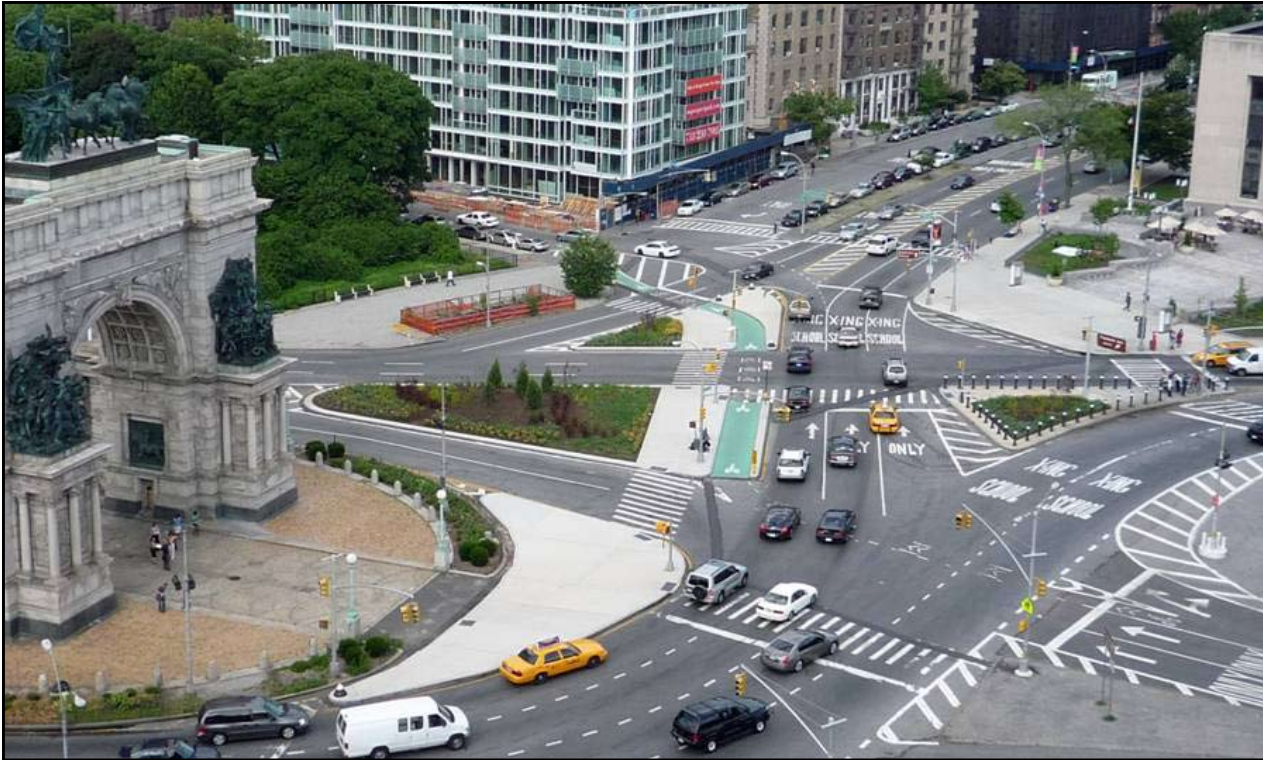
Aerial view of new pedestrian islands, plantings, and Class 1 "green" bike path
