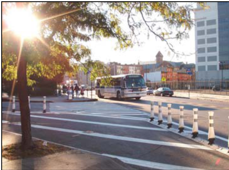
Through the use of flexible bollards and markings, the Department normalized the intersection and significantly shortened the crossing distance across Gates Avenue
