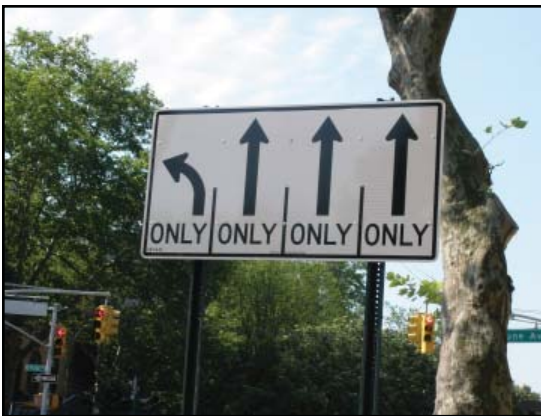
Installed new lane designation signs to more effectively direct traffic
