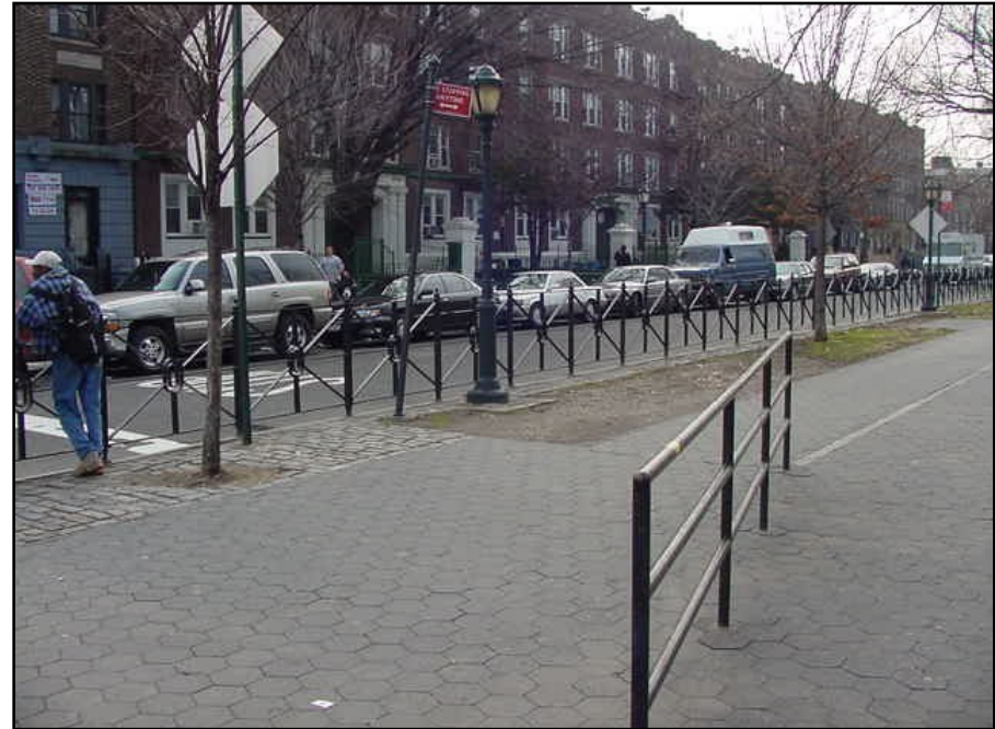
Pedestrian barriers along the service road island prevent individuals from crossing the service road midblock
