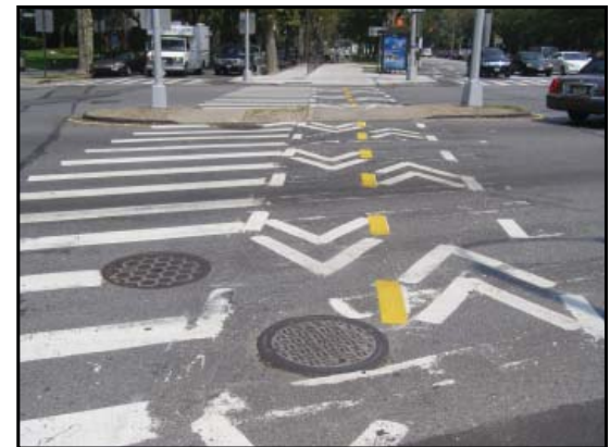
New markings between the service and main roads of Ocean Parkway direct bicycles and pedestrians and alert motorists to their presence.
