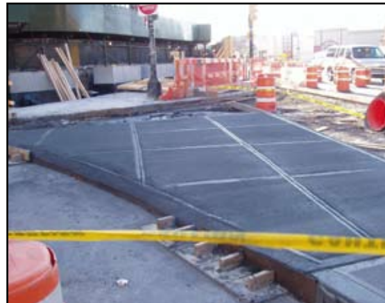
Construction phase of new pedestrian space installation
