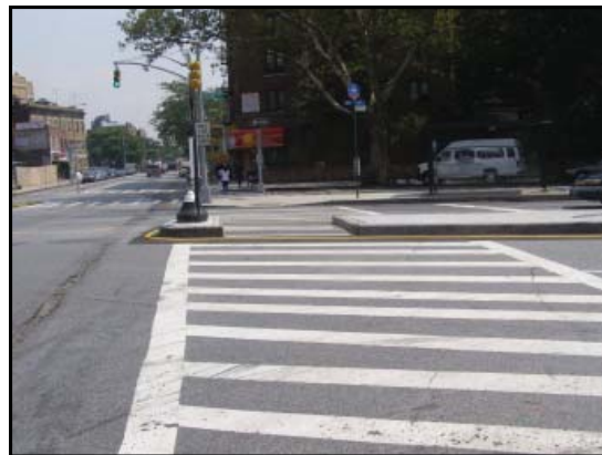
New pedestrian refuge island in south crosswalk on Ocean Parkway at Neptune Ave protects pedestrians who are unable to make it to the other side of this long crossing
