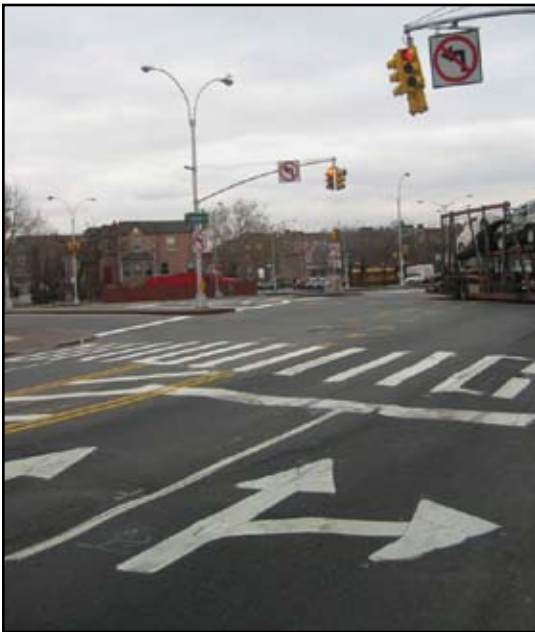
New markings and signage were installed to improve safety and operation of the intersection
