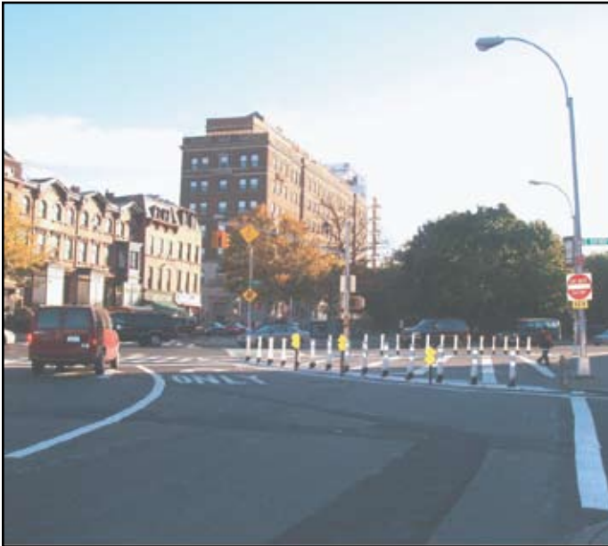
At Hanson Place, the Department eliminated the “free right turn” through the use of markings and flexible bollards, as well as shortening the crossing distance by half
