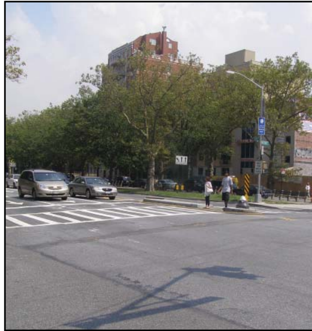
AFTER: North crosswalk on Ocean Parkway at Neptune Avenue with pedestrian refuge island
