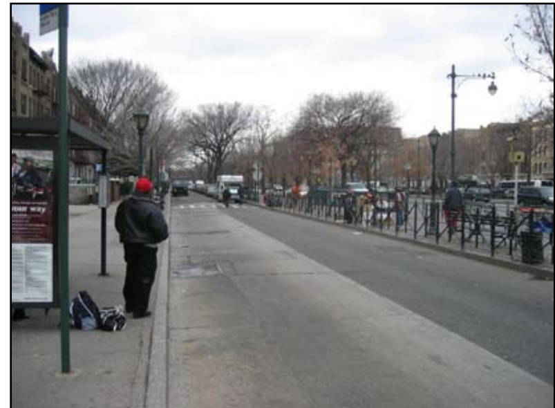
View of extended bus stop along Eastern Parkway Service Road, pedestrian barriers and additional travel lane created by removal of parking along barrier
