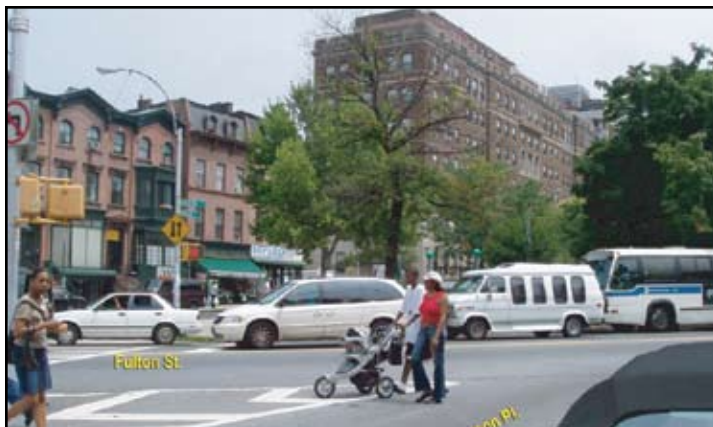
On eastbound Hanson Place approaching Fulton Street, the right-turn slip created difficult, unprotected crossing for pedestrians
