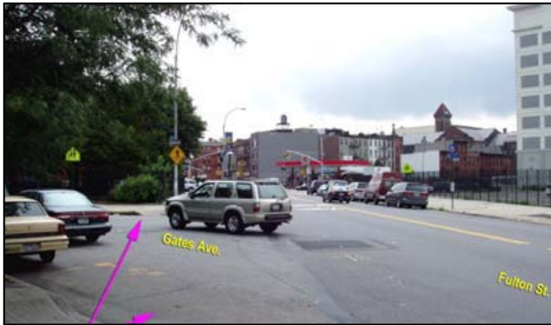
At Gates Avenue and Fulton Street, the offset geometry contributed to speeding, as well as a long crossing for pedestrians
