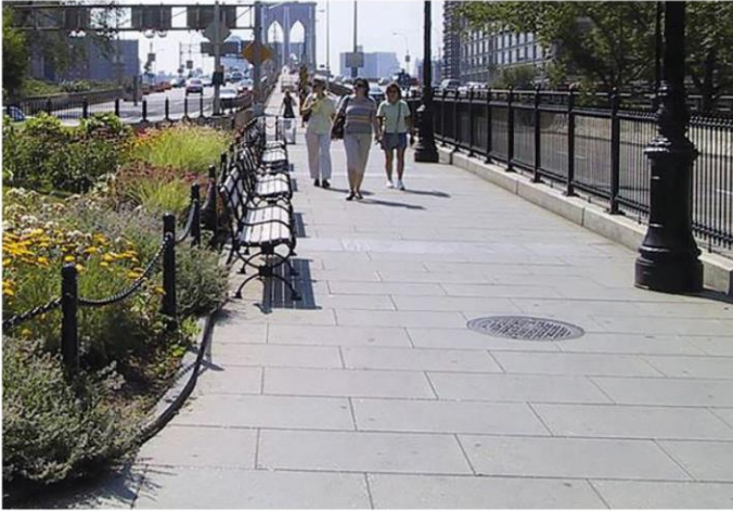
NYCDOT Concrete Pavement with London Scoring
