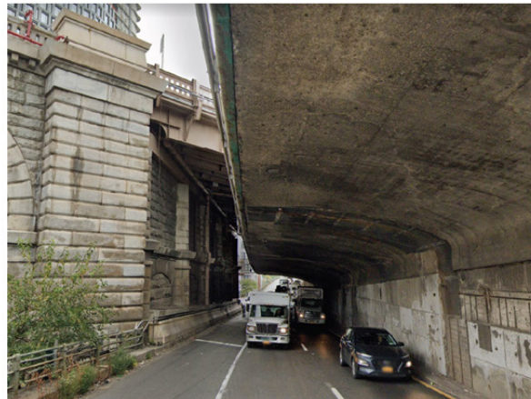
BQE Triple Cantilever at Brooklyn bridge - example of nonstandard vertical clearance
