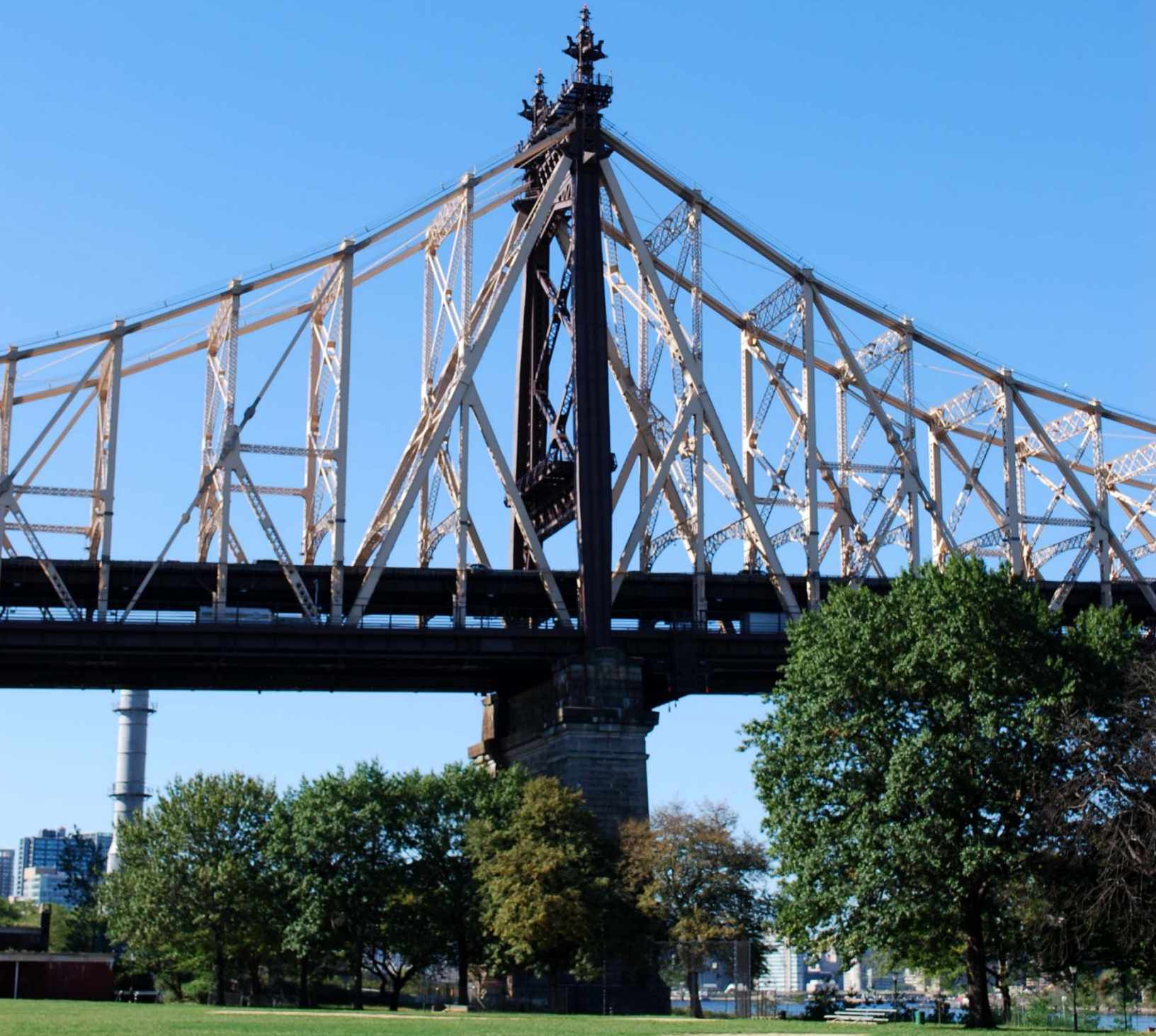
Ed Koch Queensboro Bridge
