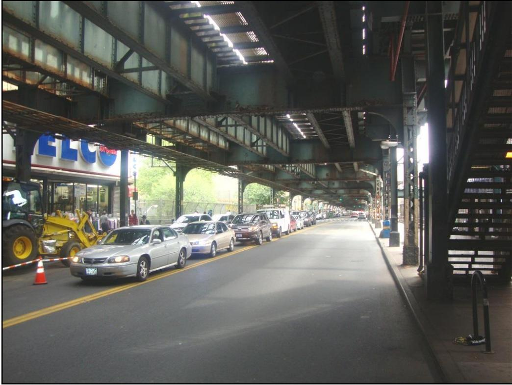
*Photograph 3: Subway Columns and Elevated Subway Structure*
