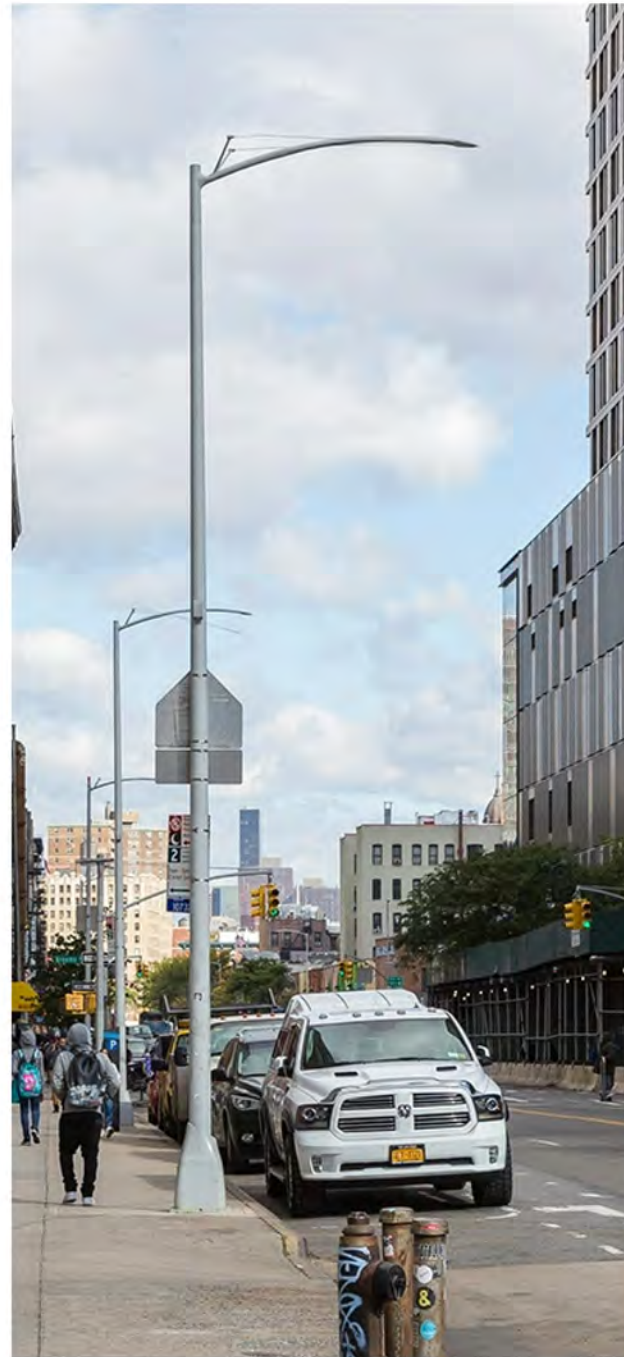
Street light fixture - City Light
