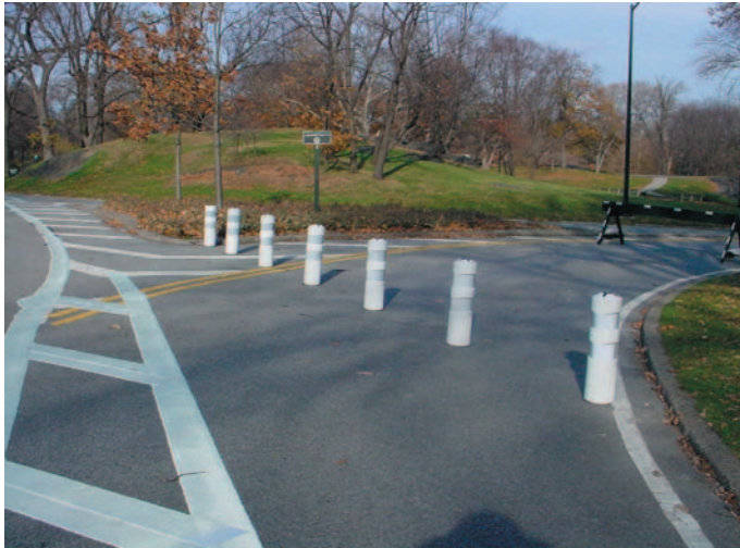
West 72 nd Street Slip-Off Ramp Closure
