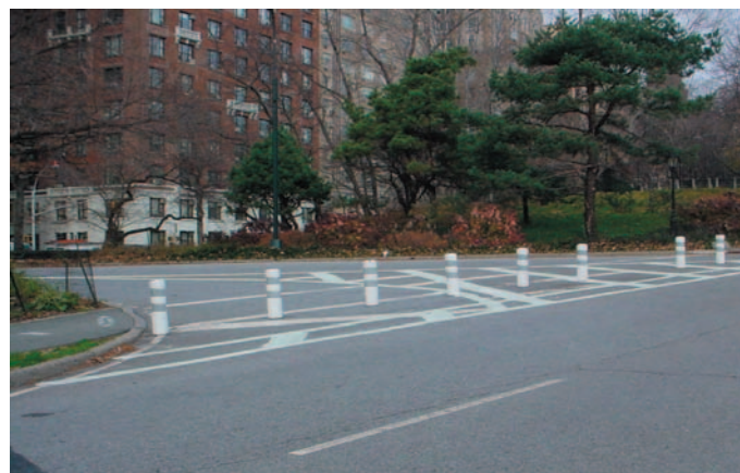
West 90 th Street Exit Closure
