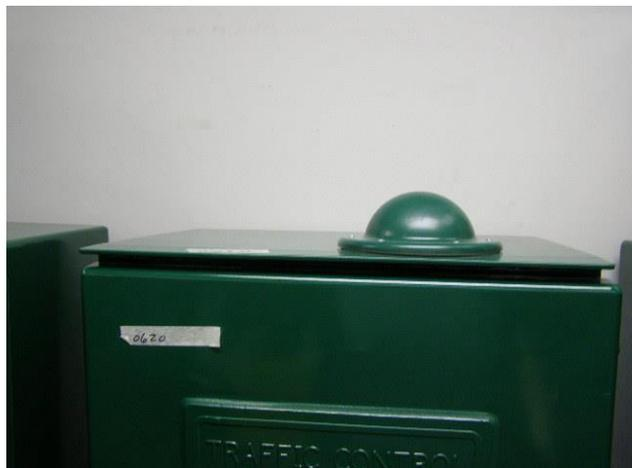
48.2.2. A hole  $\frac{7}{8}$ " is drilled in the top of the cabinet. The antenna is seal against water leakage into the cabinet using a bead of silicon to the underside of the antenna before installation the antenna is secured by tightening the nut on the mounting stud of the antenna once the mounting stud is passed though the  $\frac{7}{8}$ " hole in the cabinet top.
