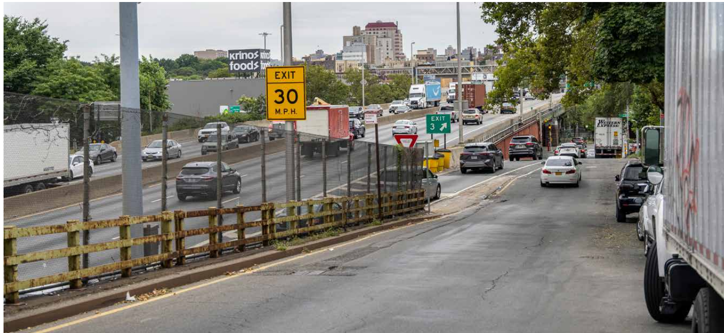
Figure 5.1 Cross Bronx Expressway at Arthur Avenue and East 175 th Street
