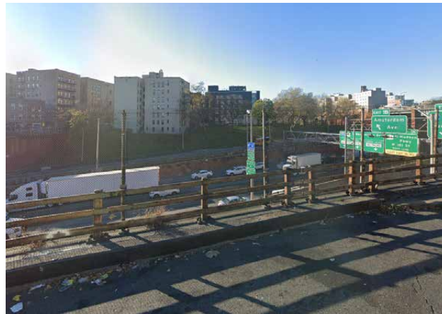
Figure 4.23 View South from Plimpton Avenue
