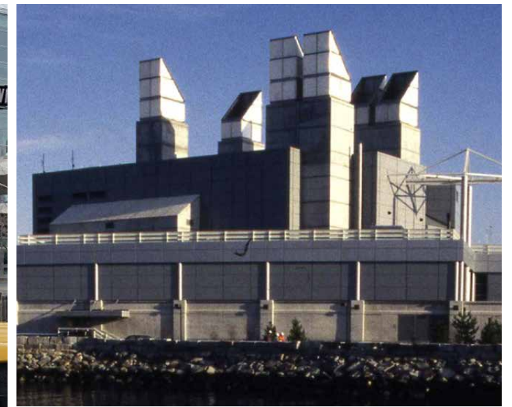
Figure 4.42 Ventilation Building No. 6 for the Central Artery in Boston
