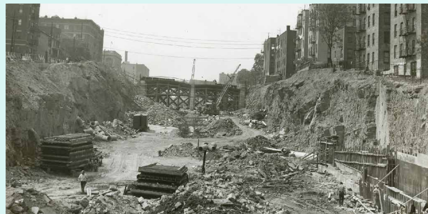
Figure 2.2 Cross Bronx Expressway under construction in 1948. Source: Lehan College Library (CUNY)
