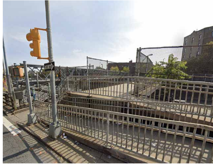
Figure 4.46 Existing Condition of Olmstead Avenue Footbridge
