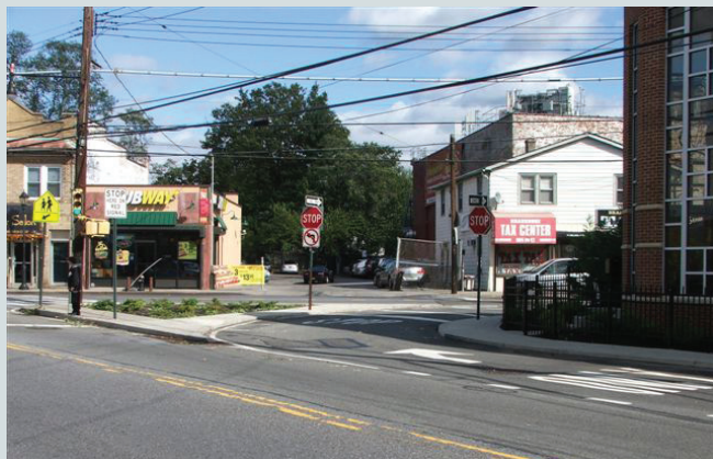
A channelized right-turn lane was constructed at Nelson Avenue for eastbound Amboy Road traffic to help calm traffic.
