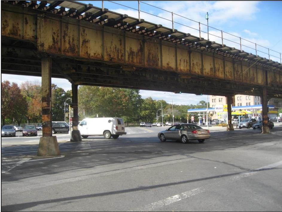
*Figure 18: White Plains Road at Bronxdale Road intersection (Before Condition) - Worn-out paint on subway columns and subway steel structure*
