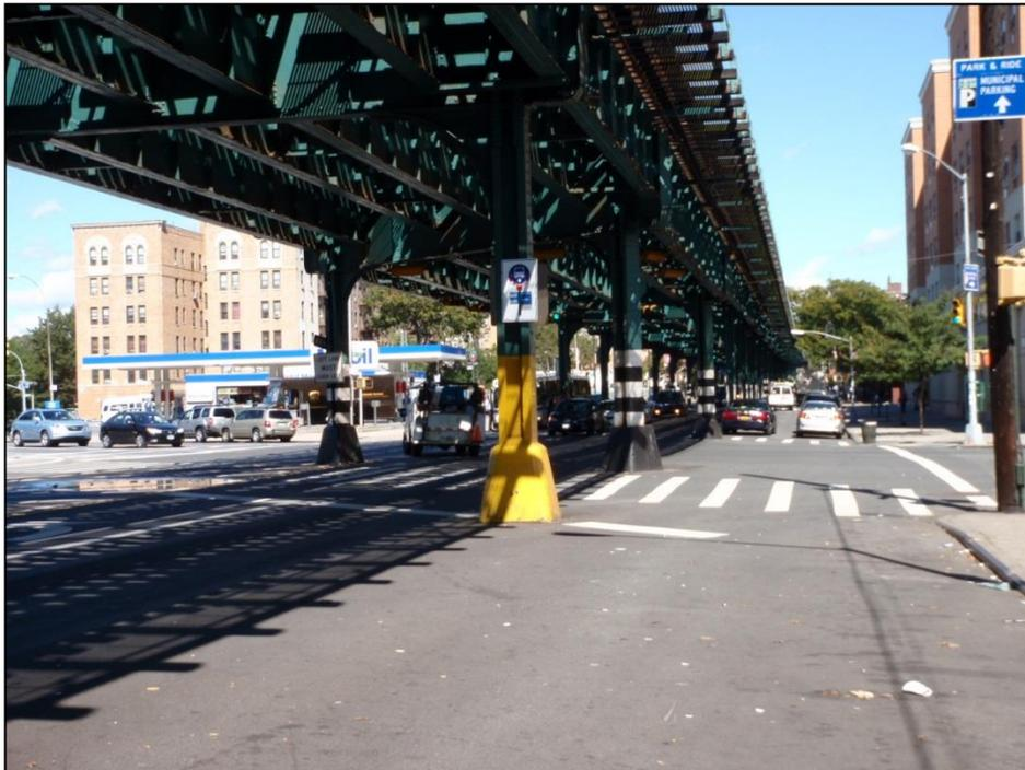
*Figure 19: White Plains Road at Bronxdale Road intersection (After Condition) - New paint applied on subway columns and subway steel structure in 2011/2012 for positive delineation and safer traffic operations*
