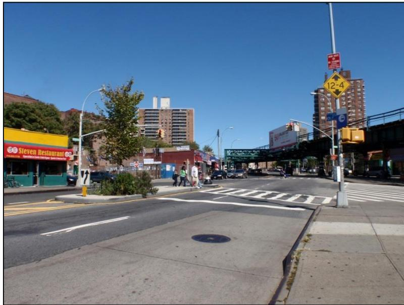
*Figure 32: New median island installed at south side of Boston Road and Thwaites Place intersection*
