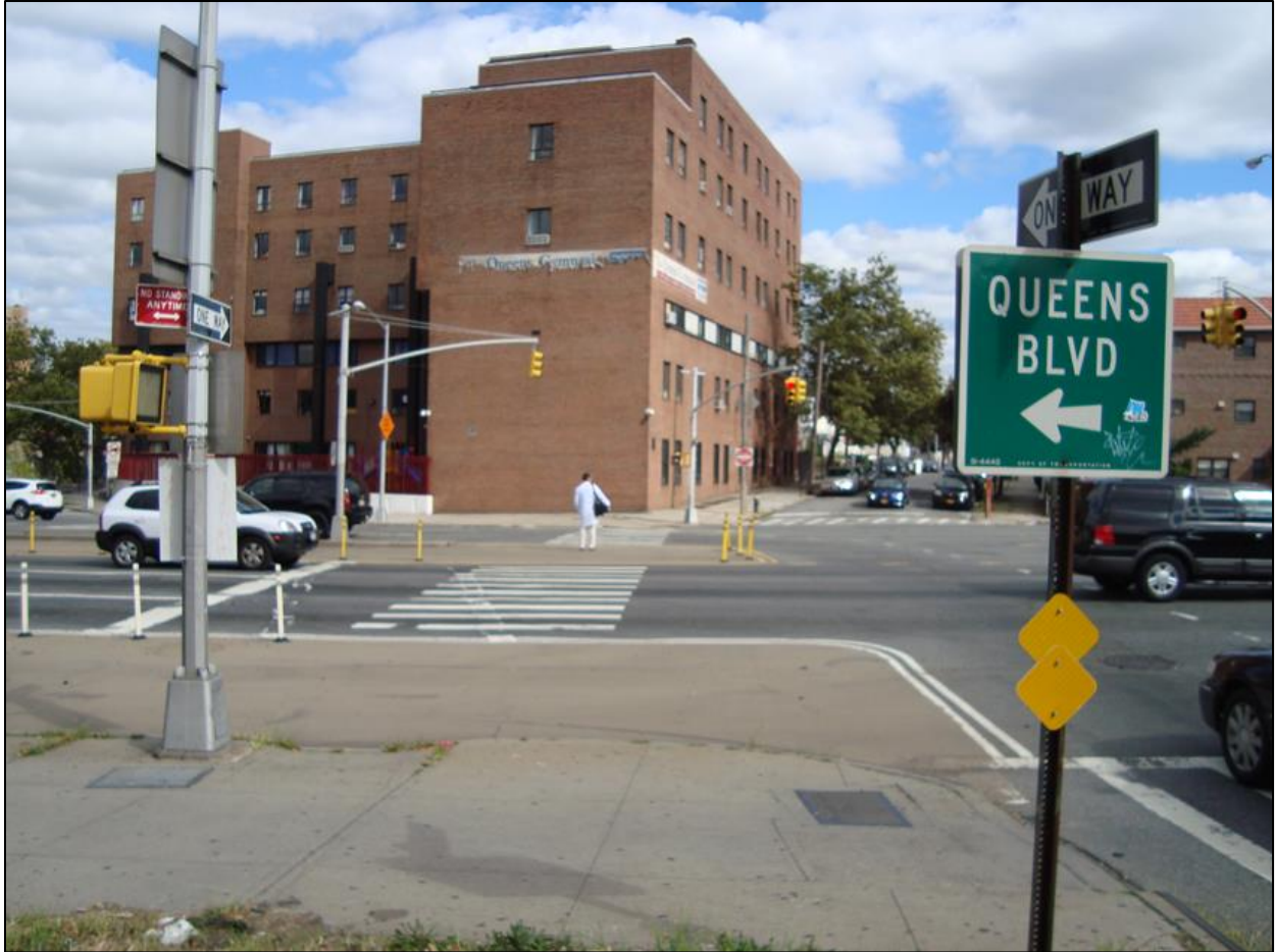
Photo 3.2-1: North crosswalk, median refuge and curb extension, at Wetherole Street
