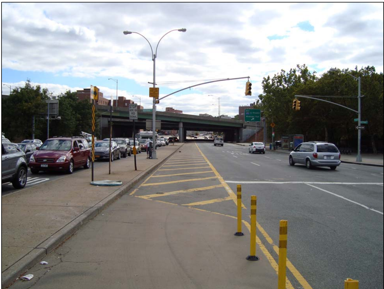
Photo 3.1-4: Left lane of Southbound Woodhaven Boulevard removed with diagonal striping
