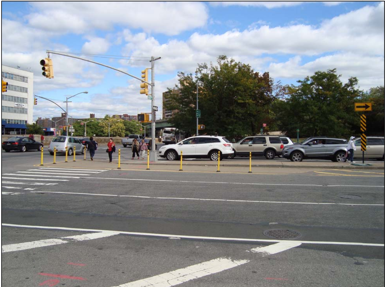
Photo 3.1-2: Widened median, south crosswalk, at Queens Boulevard
