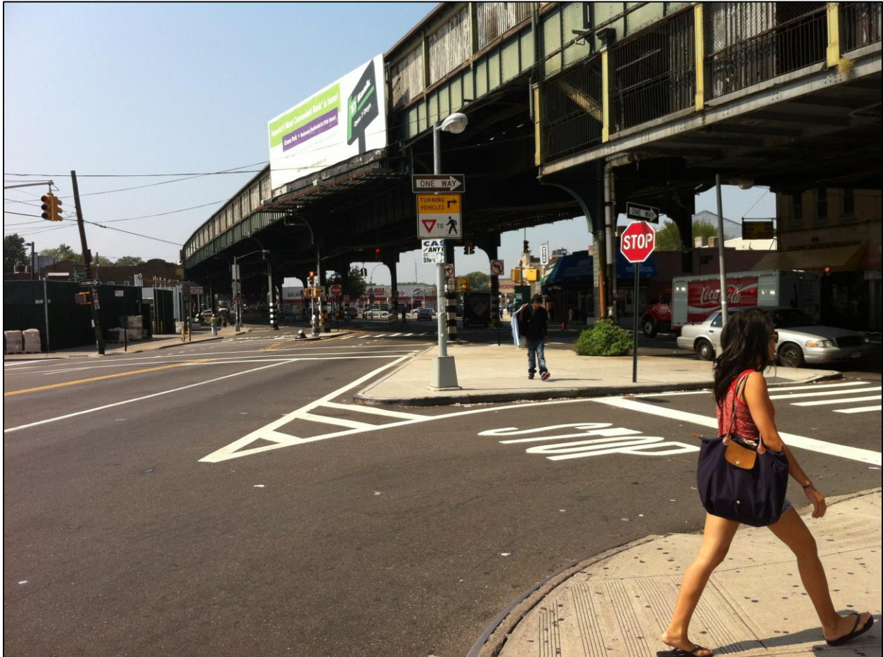
Photo 3.8-3: New pedestrian refuge island along the east side of 96 th Street at the Liberty Avenue/Rockaway Boulevard junction
