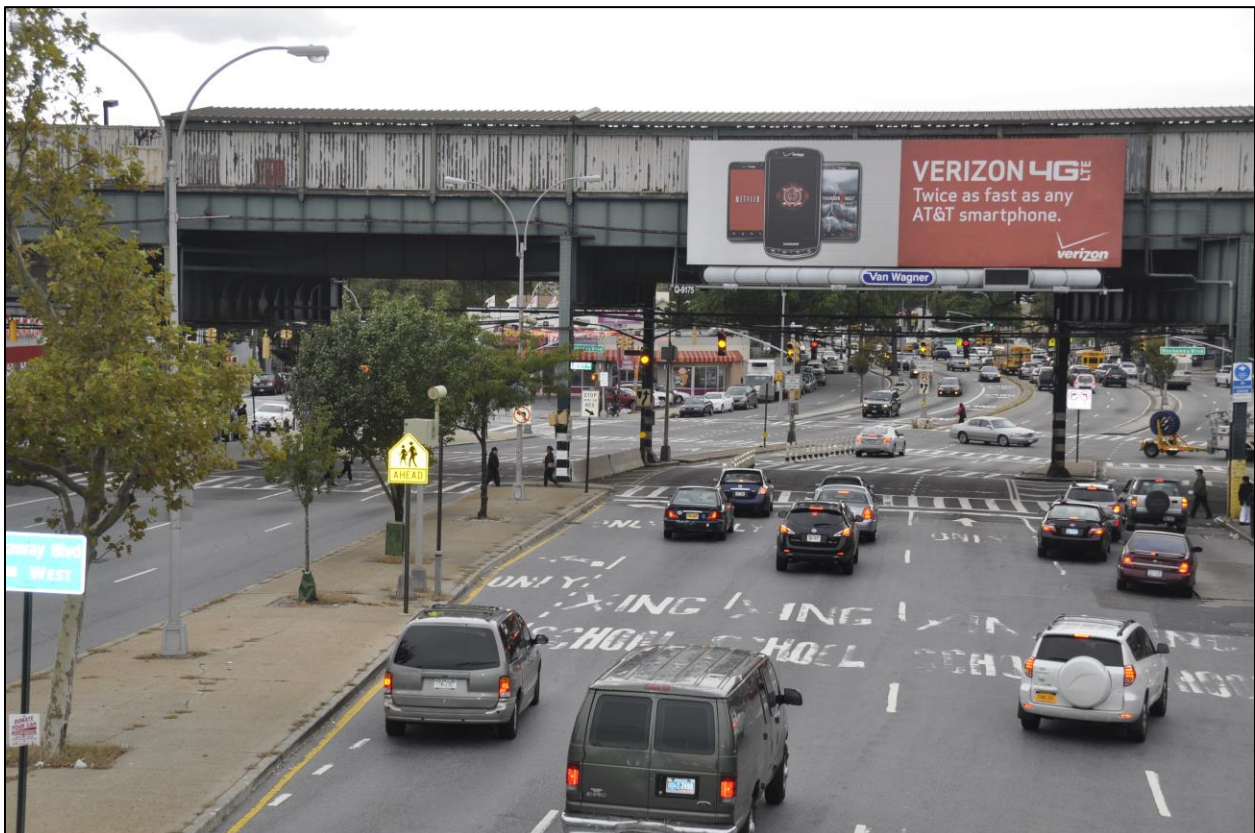
Photo 3.8-1: Crossbay Boulevard looking north towards Liberty Avenue
