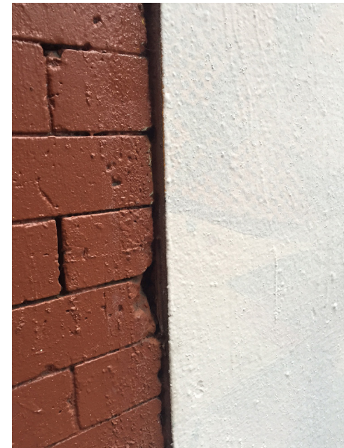
Current Condition - close up
