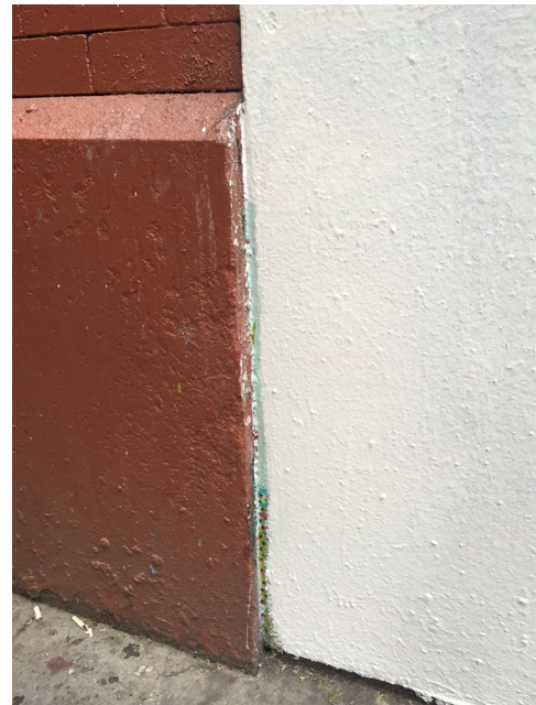
Current Condition - close up
