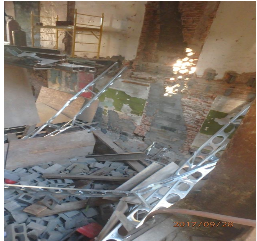
Overloaded Metal Deck
