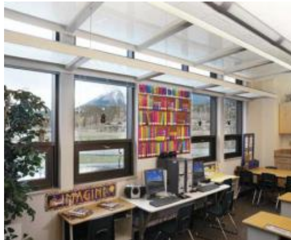
Figure LE-5.b. Daylight zone with automatic controls Exempt from Light-Reduction Controls Source: energycodes.gov/training
