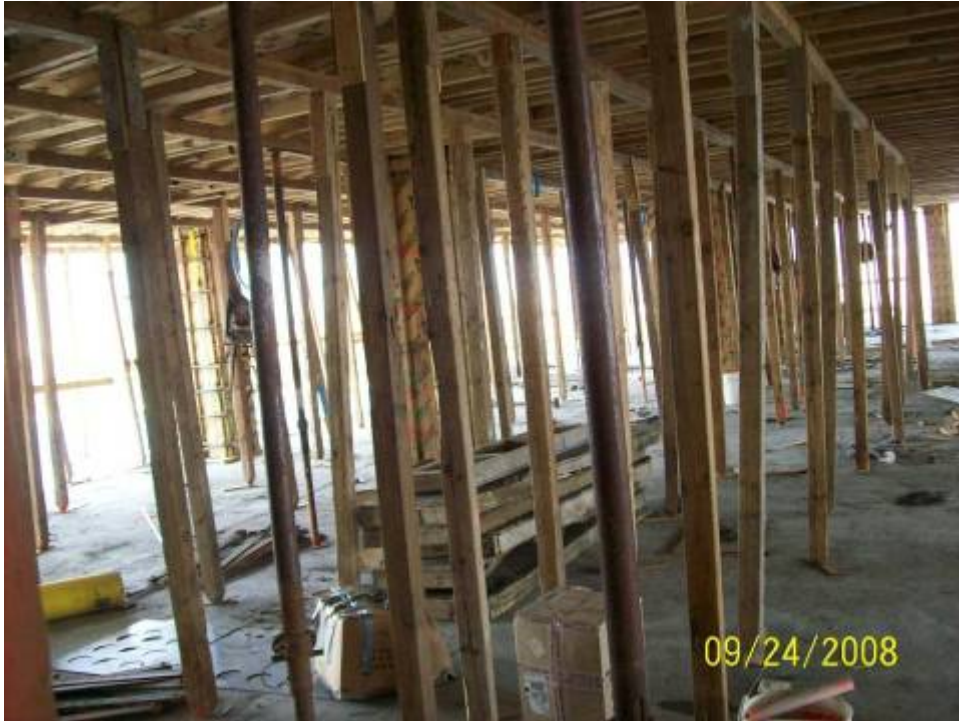
Figure B.6.1: Typical Stick Formwork Assembly consisting of Timber Posts and Lumber Framing Elements
