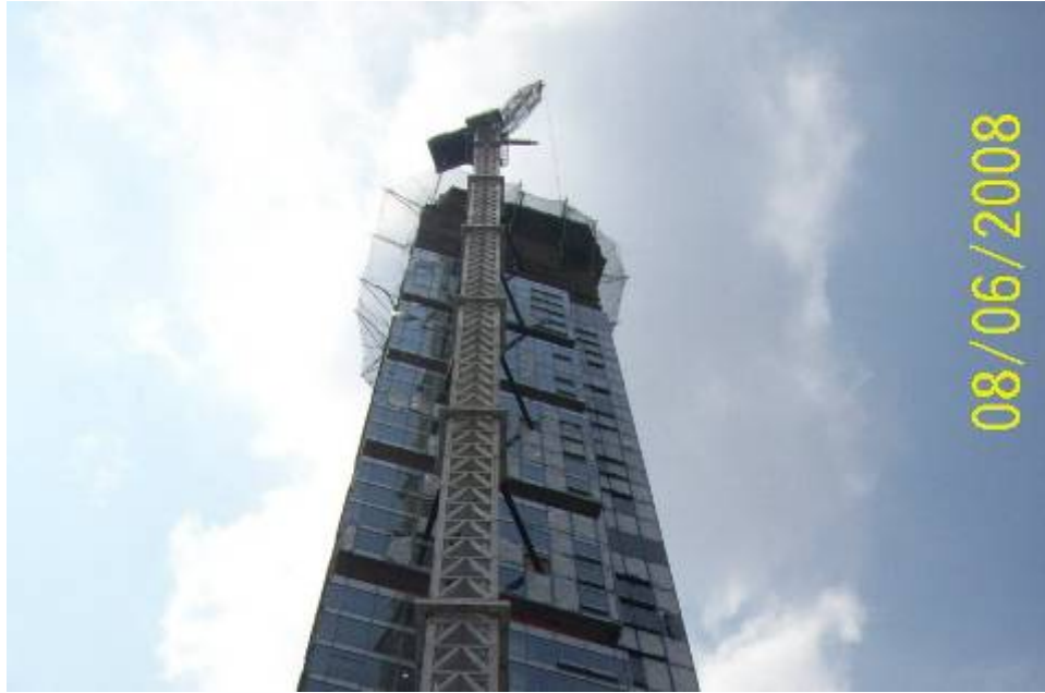
Figure B.7.15: Cocoon Construction in Operation.
