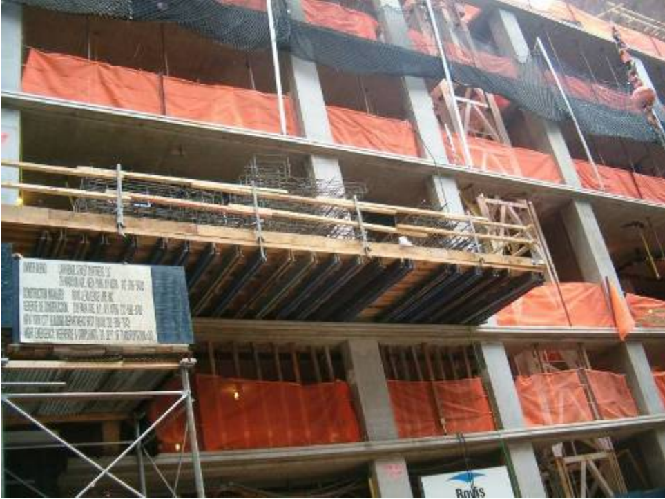
Figure B.7.16: Acceptable Outrigger System for Material Handling Near Ground Level. Note Uninterrupted Edge Protection.
