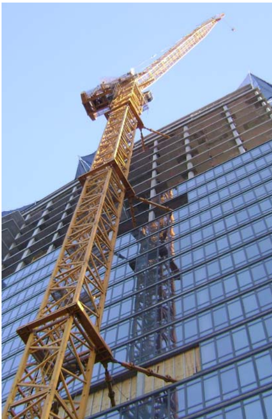
Figure C.7.1: Examples of Tie-ins (Site C-10)
