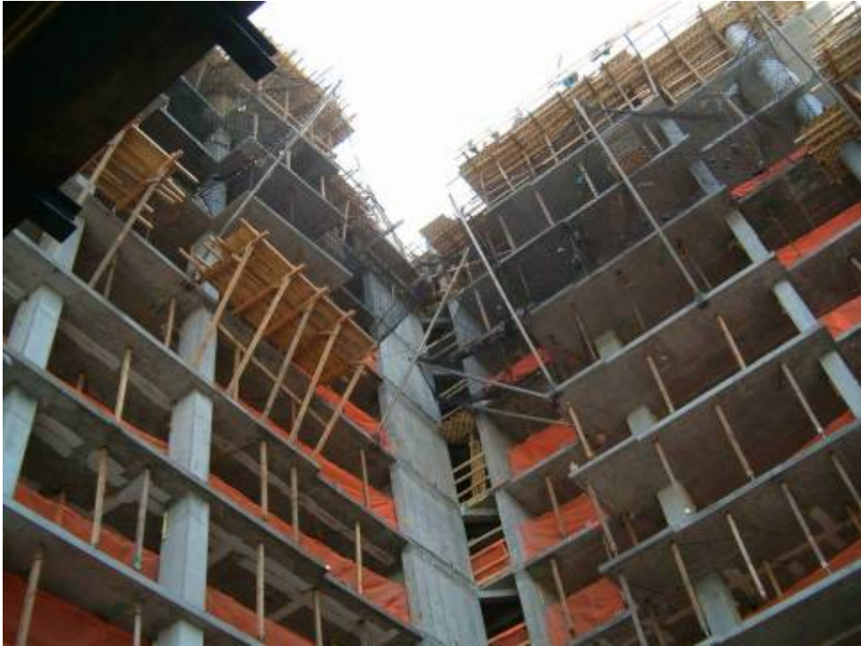
Figure B.7.6: Building Exposure with Incomplete Edge Protection. Code Provisions Do Not Address Violation Thresholds Relating to Percentage of Exposure without Protection
