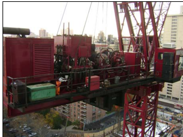
Figure C.6.8: Diesel Hydraulic Crane
