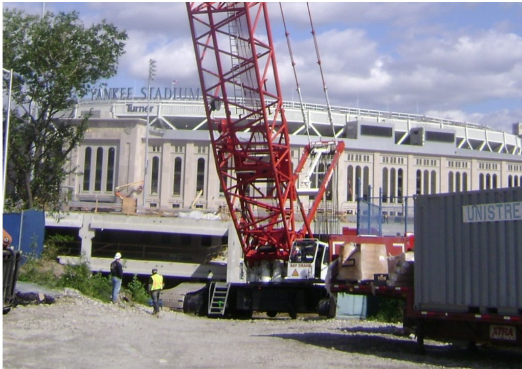
Figure C.9.12: Crane Observed During CN “Sweep”
