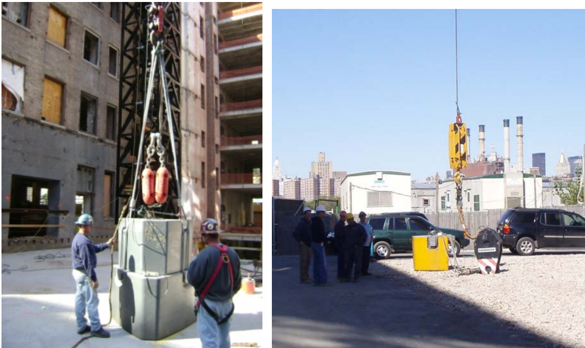
Figure C.7.13: Load Test in Operation
