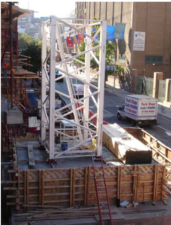
Figure C.7.8: Tower Crane Foundation (Site C-3, 9/5/08)
