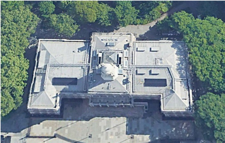
City Hall City Hall Park, New York, NY 10007 Completed April 2015 10.4 kW
