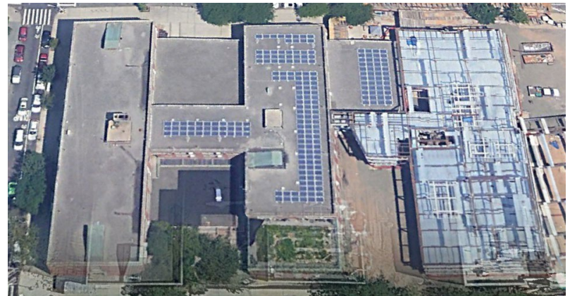
Brooklyn Repair - Remsen Yard 855 Remsen Ave Brooklyn, NY 11236 Completed January 2011 43.52 kW (Thin Film)
