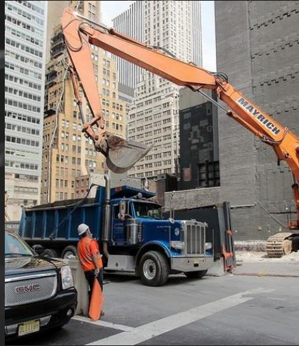
Construction & Demolition Debris
