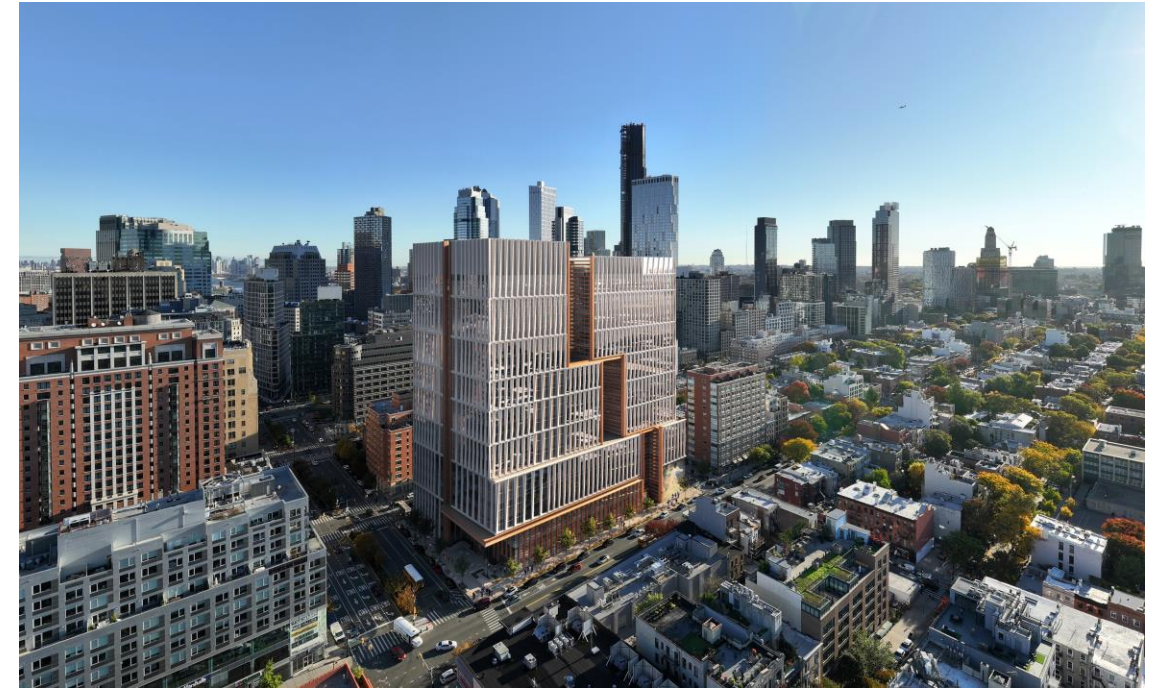
Aerial View from Southwest
