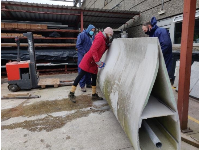
Re-Wind BladeBridge, cutting blade to build pedestrian bridge
