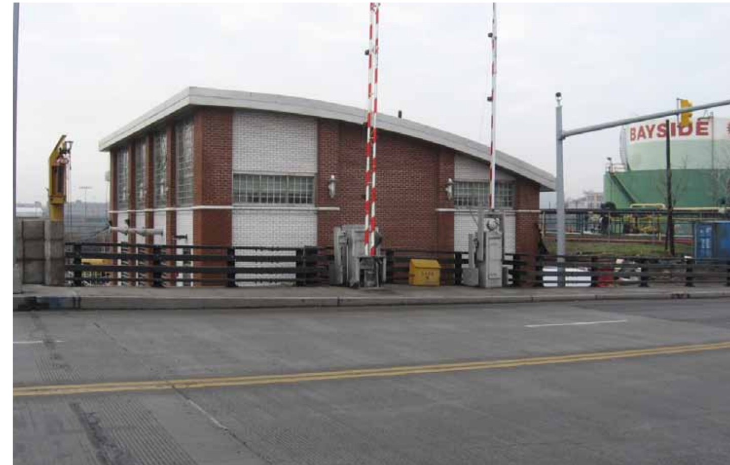
English Kills In-Stream Aeration
