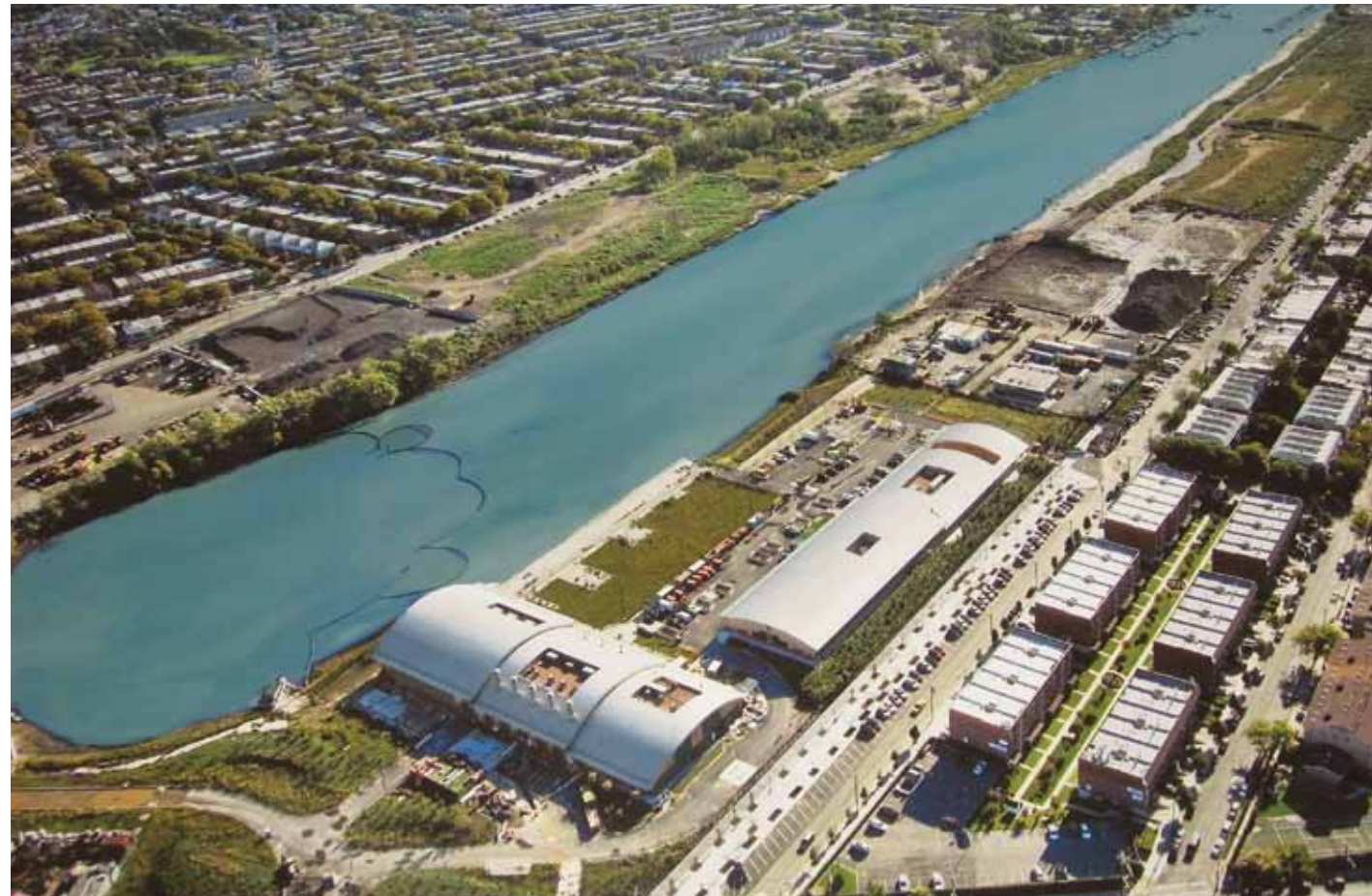
Paerdegat Basin CSO Retention Facility
