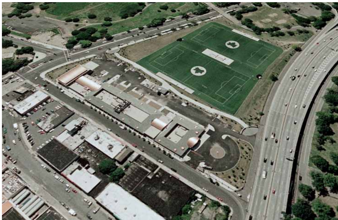
Flushing Bay CSO Retention Facility
