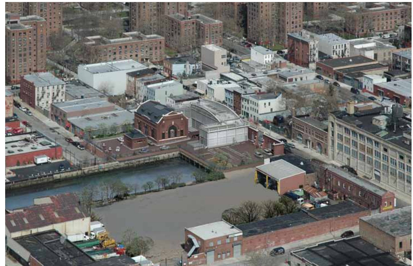
Gowanus Canal Pump Station & Flushing Tunnel
