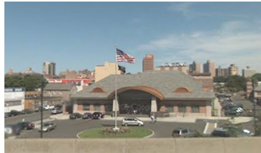
Flushing Bay CSO Retention Facility
