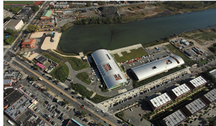
Paerdegat Basin CSO Retention Facility
