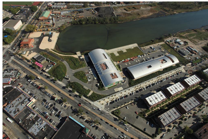
Paerdegat Basin CSO Retention Facility
