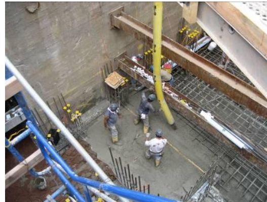
Pump Station Expansion
