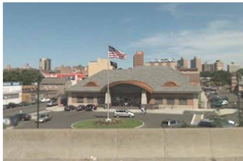
Flushing Bay CSO Retention Facility
