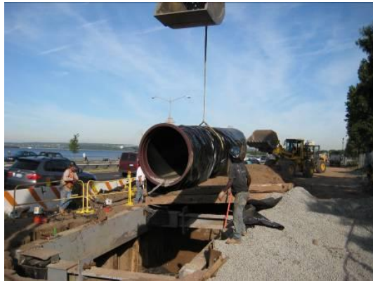
New Sewer Construction
