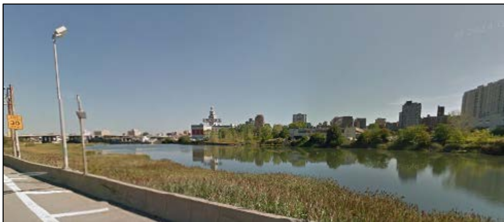
Figure 2b. Flushing Creek Shoreline (Looking Northeast from Van Wyck Expressway)
