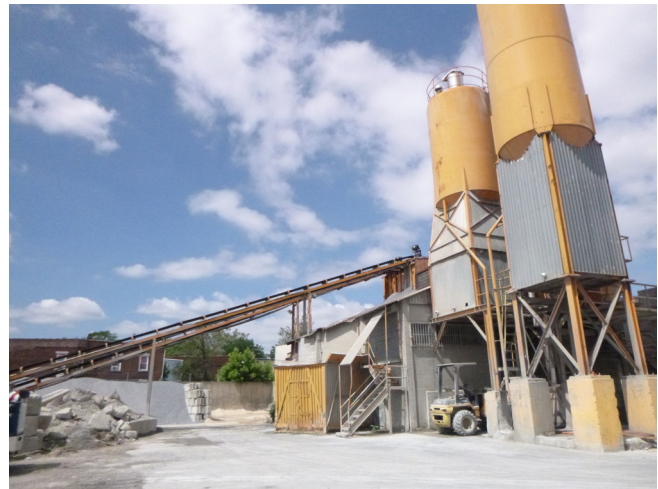
DEP and Stantec inspected MSGP permitted sites, such as this concrete manufacturing facility.
