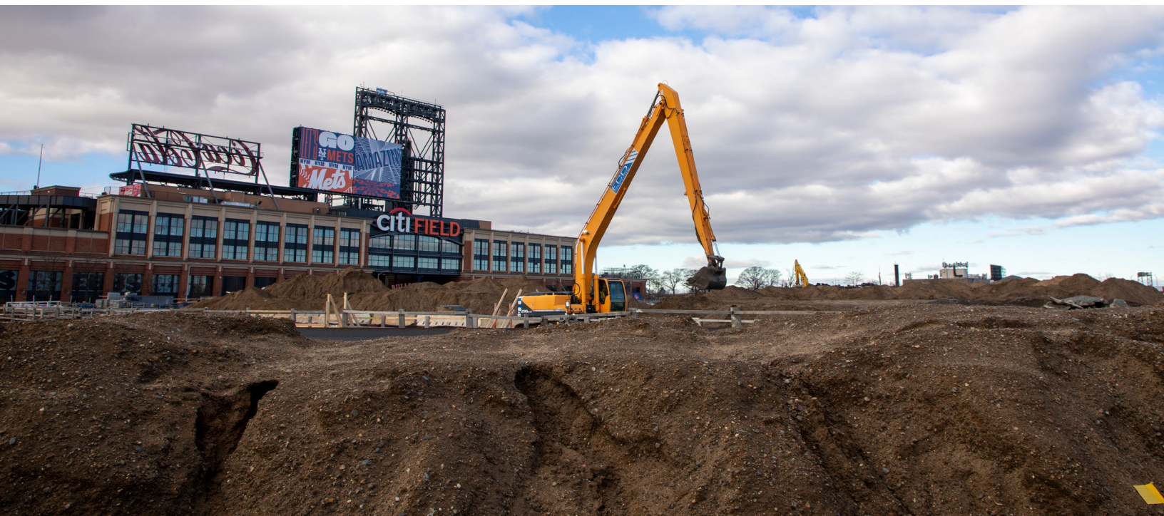
Willets Point construction progress.
